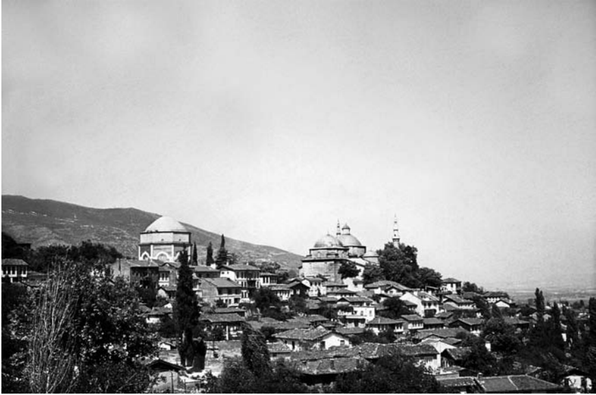
FIGURE 8.1 Bursa, zāviye/‘imāret and complex of Meḥmed I, the “Green Mosque,” 822/1419 BY PERMISSION OF THE BOĞAZIÇI UNIVERSITY APTULLAH KURAN ARCHIVE
