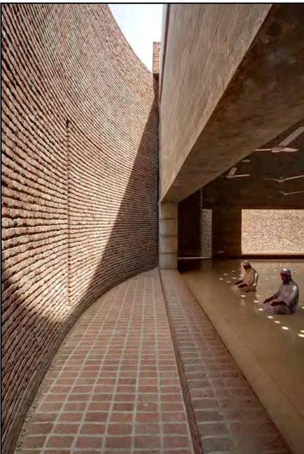
The monsoon rain may pose a problem as the openings for the hot air to escape also allow in rain. However, it is important to keep cross-ventilation even when it is raining, and the rain seems to have good drainage in the spaces where it enters.
