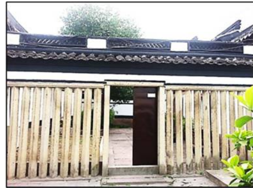
Figure 9. The Northern wall of Eastern courtyard
