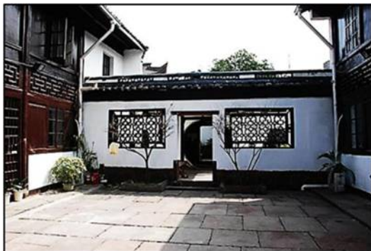
Figure 14. General view of the western courtyard
