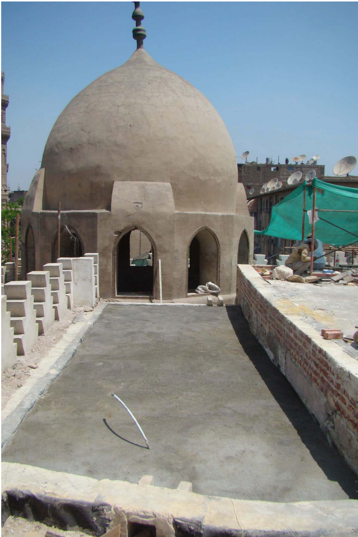
Roofing work in progress
