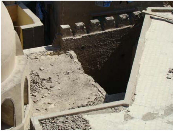
General view showing the existing condition
