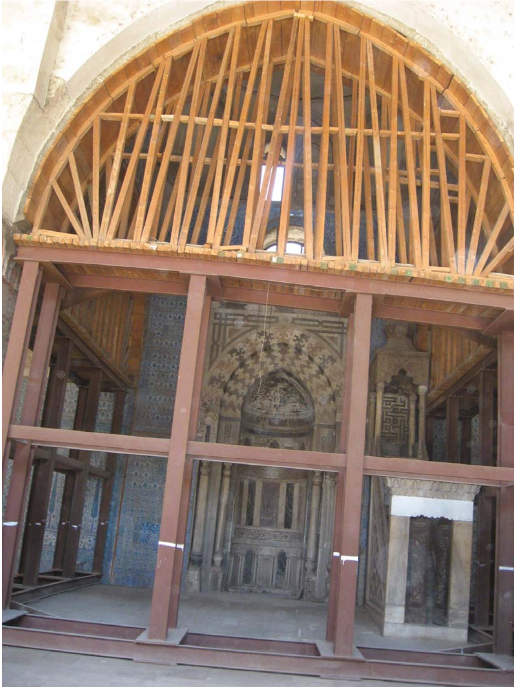
Picture A1: Steel shoring for the courtyard arches.
