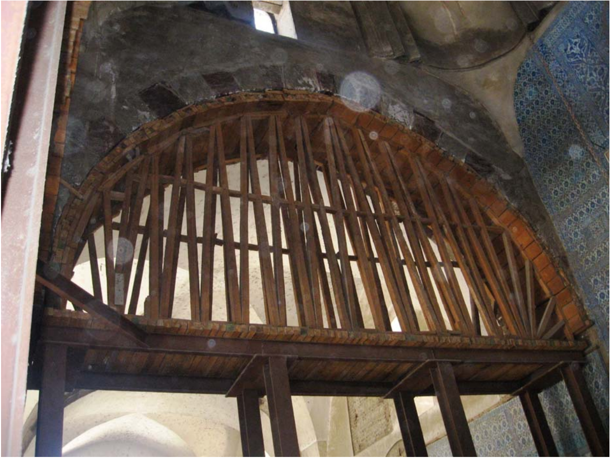
Picture A2: Details of contact between shoring and arches.
