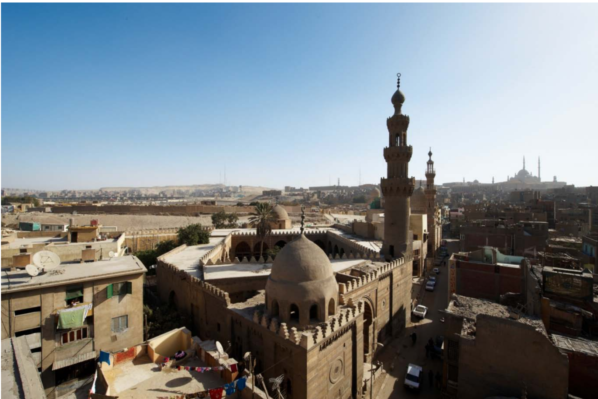
General view of the building from the North-East, including Kujuk mausoleum in the foreground, the minaret (of which the top fragment was reconstructed in 1924) and in the background the mosque's courtyard and cupola over the covered prayer area. The building is aligned on darb al-Ahmar Street leading to the Citadel, centre of sultanate power.
