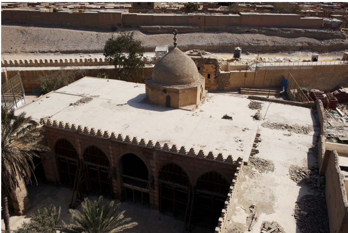
(Top) General view of the roofs covering the prayer area: roofing system is made by parts and not fully leveled to ensure proper rain water drainage. Decayed materials accumulate in several areas.
