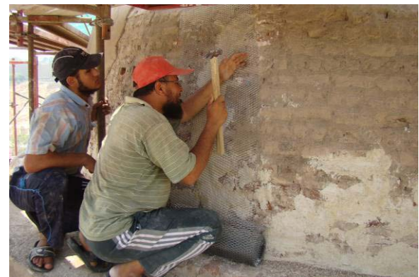
Installing the galvanized steel mesh
