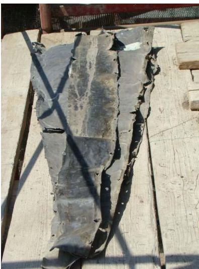
View of the old led sheets
