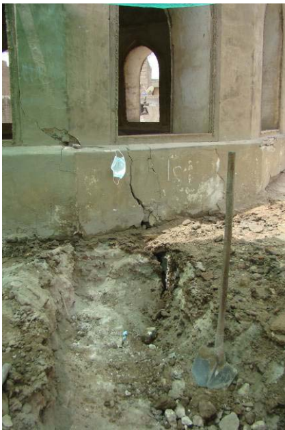
Crack repair in the drum of the dome
