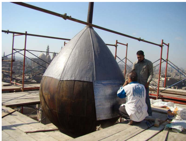
View of the wooden bulb during the led sheets installation
