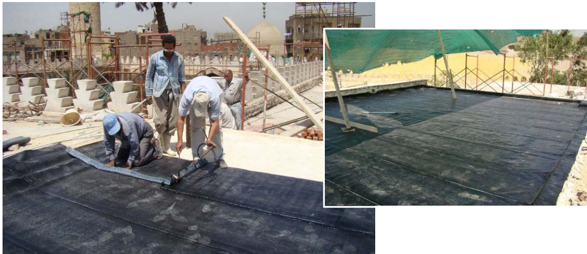
Application of the bitumen sheets for water insulation
