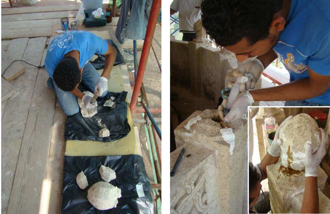
Fixing and Assembling process of the stone column top
