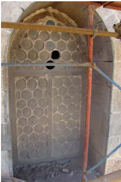
Dismantling the mesh windows
