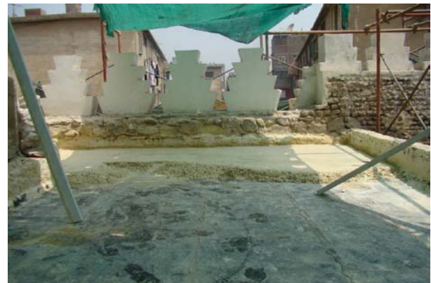
Final mortar application on top of water insulation
