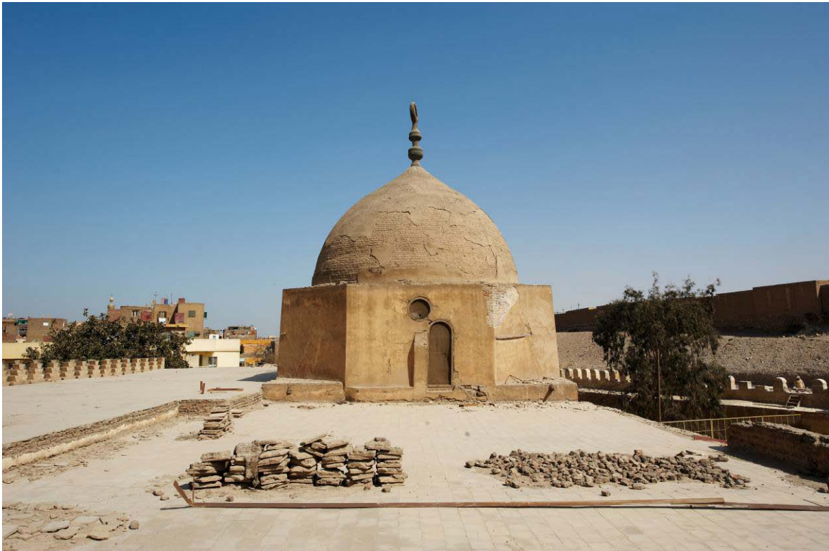
View of the qibla dome before starting the restoration & conservation
