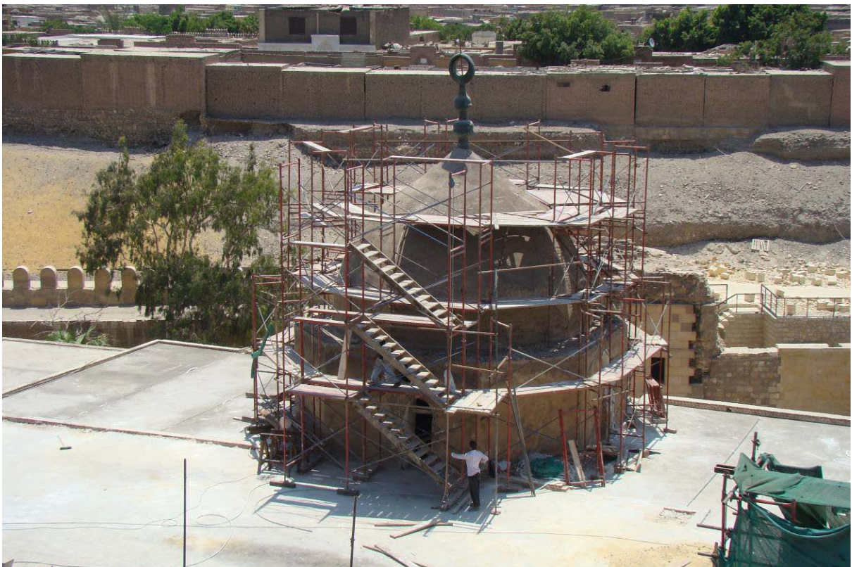
View of the qibla dome after erecting the scaffolding
