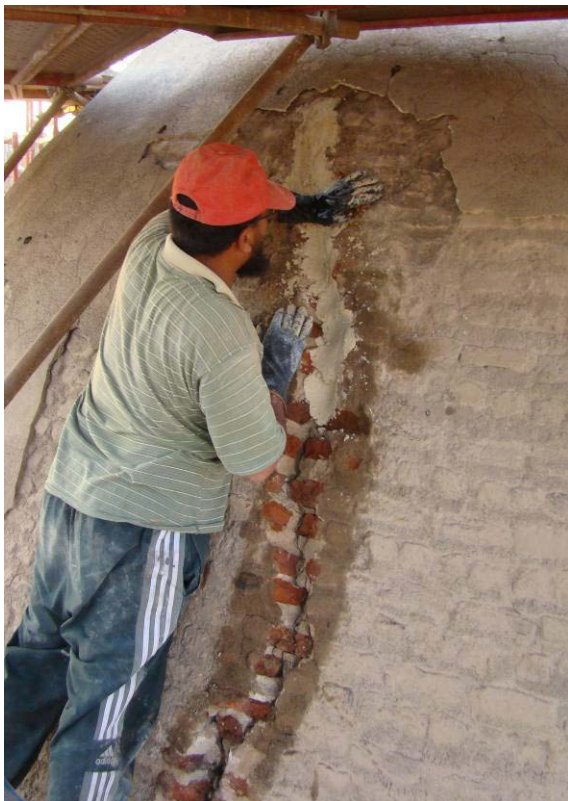
Filling the vertical cracks
