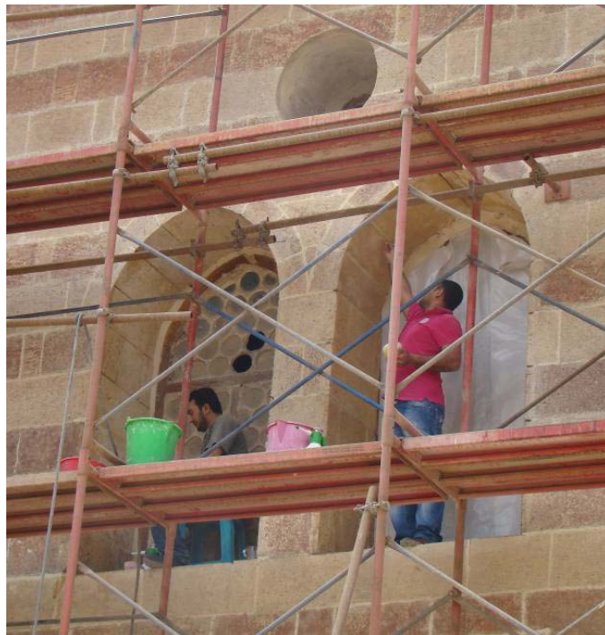
Conservation and cleaning activities of the stone openings
