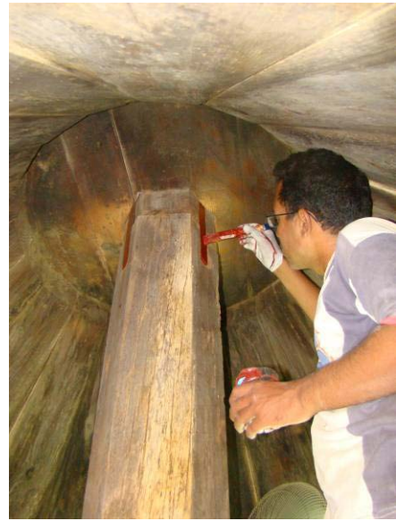
Cleaning of the interior and insulation of metal
