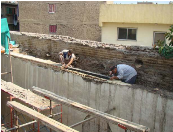
Installation of wooden cushions along the side walls
