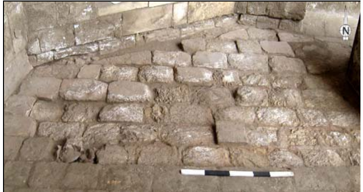
doc. 14 : TP2 : Pavement after its cleaning
