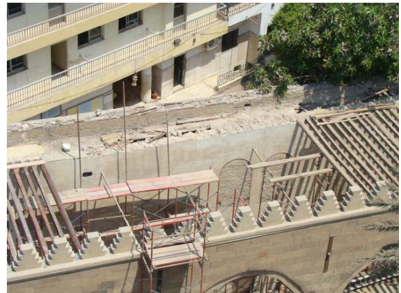
View of the roof
