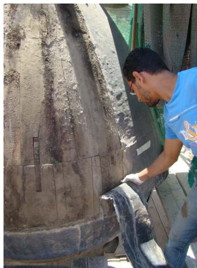
Dismantling of the led sheets
