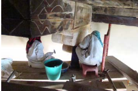
Cleaning and conservation activities using soft brushes, water & alcohol
