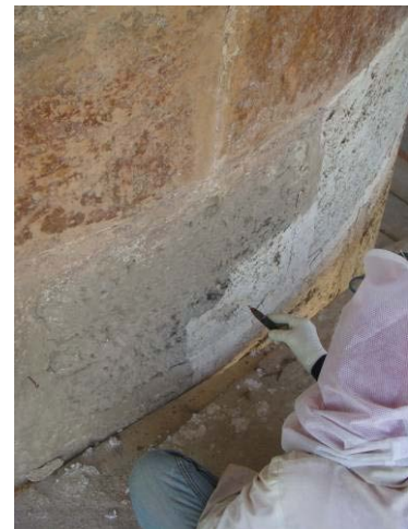
Micro-sand blasting of the lower stone body
