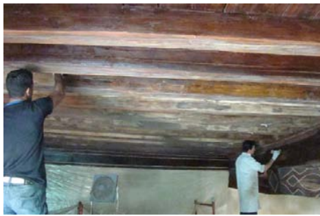
Painting the non-decorative beams
