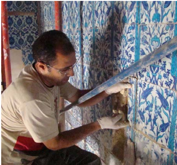
The conservation and re-touching activities of the mausoleum's entrance
