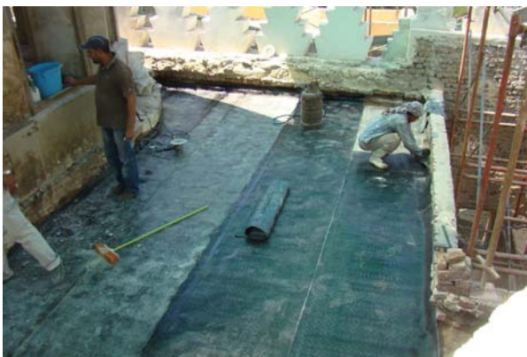
Application of insulation sheets
