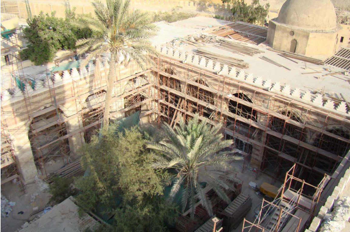
View of the courtyard facades with site installations and scaffolding
