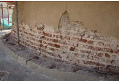
View of the lower part after removing the plaster
