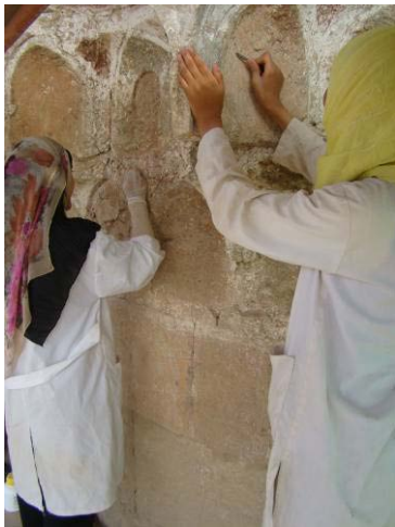
Mechanical cleaning of the lower balcony stalactites
