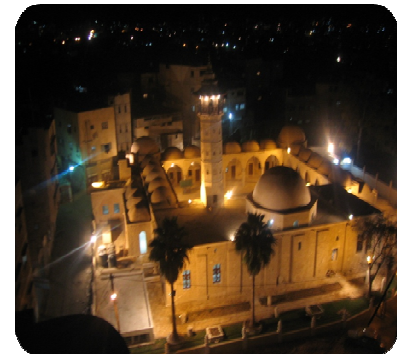
Figure 3: Photo of the mosque after rehabilitation
