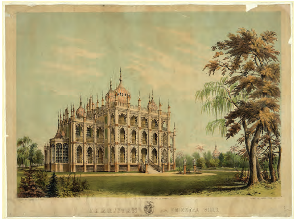
Fig.3.2 Leopold Eidlitz (architect), Iranistan, Bridgeport, Connecticut, USA. 1848. Library of Congress, Prints & Photographs Division, Washington, DC., LC-DIG-pga-04090.
