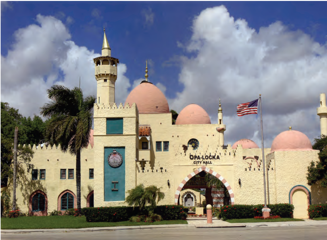
FIGURE 3.5 Bernhardt Muller (architect) and Glenn H. Curtiss (developer), Opa Locka City Hall, Miami, Florida, USA. 1929. Photo: Phil Pasquini.
