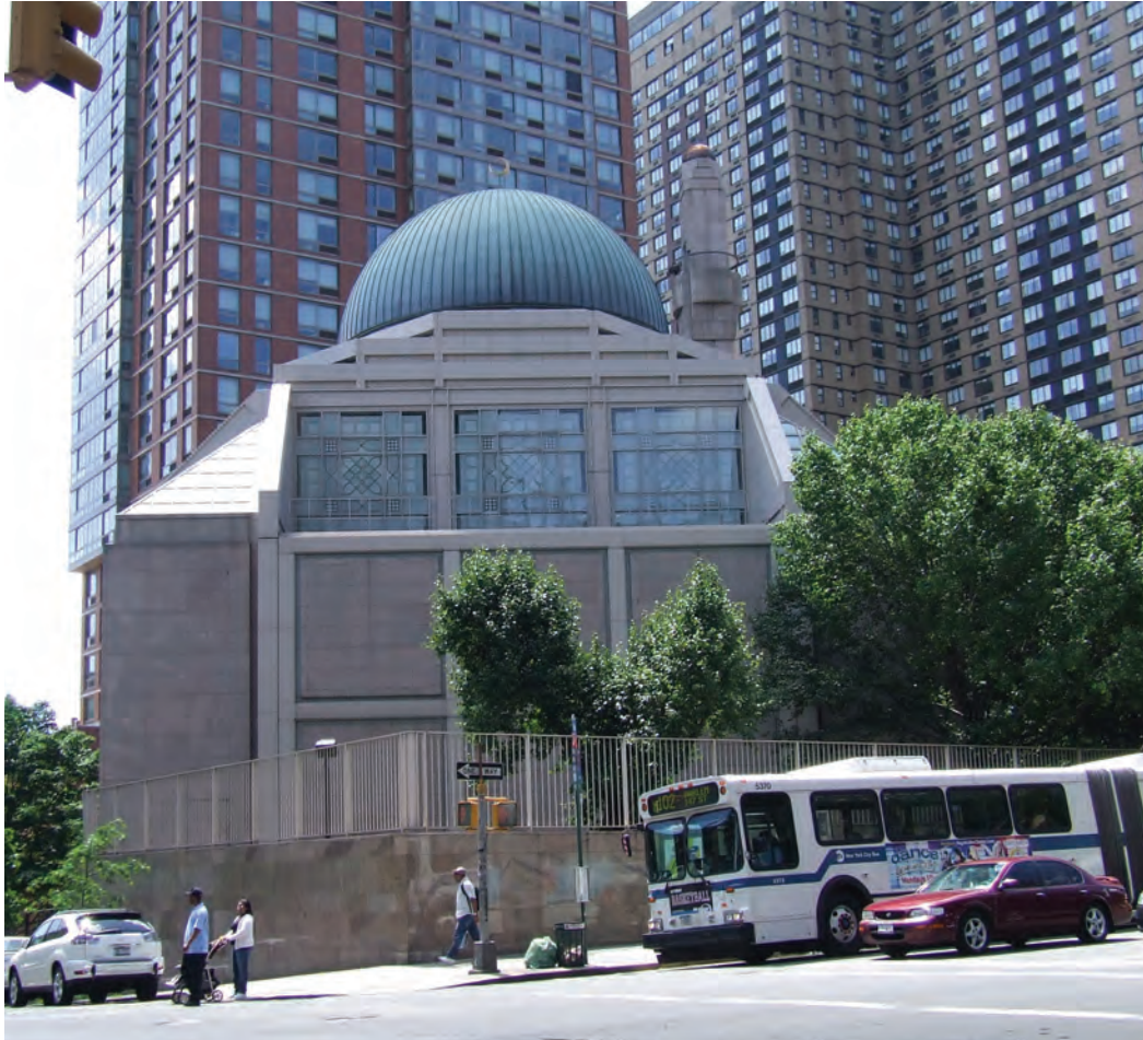
Fig 4.14 Skidmore, Owings and Merrill (architects), Islamic Cultural Centre of Manhattan, New York, USA. 1986-1991. Photo: Nadia Kurd, 2009.
