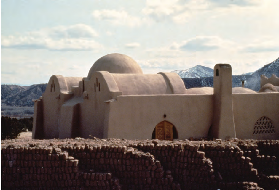
Fig 4.19 Hassan Fathy (architect) Dar al Islam Mosque and complex. Abiquiu, New Mexico, USA. 1980. Photo: Omar Khalidi, c. 1980s.
