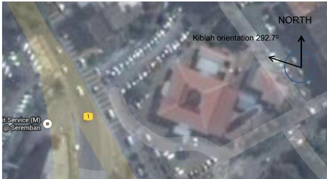
Figure 4. 8 - The aerial view of Jamek Mosque, Seremban (from Google Map)
