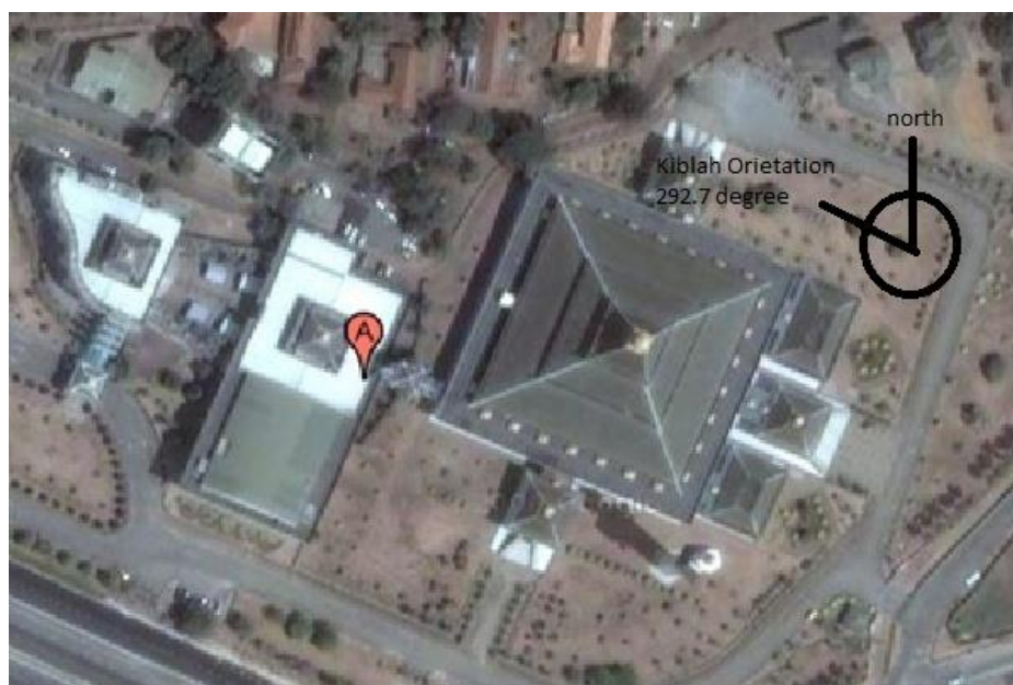
Figure 4. 4 - The aerial view of the mosque (Google map)
