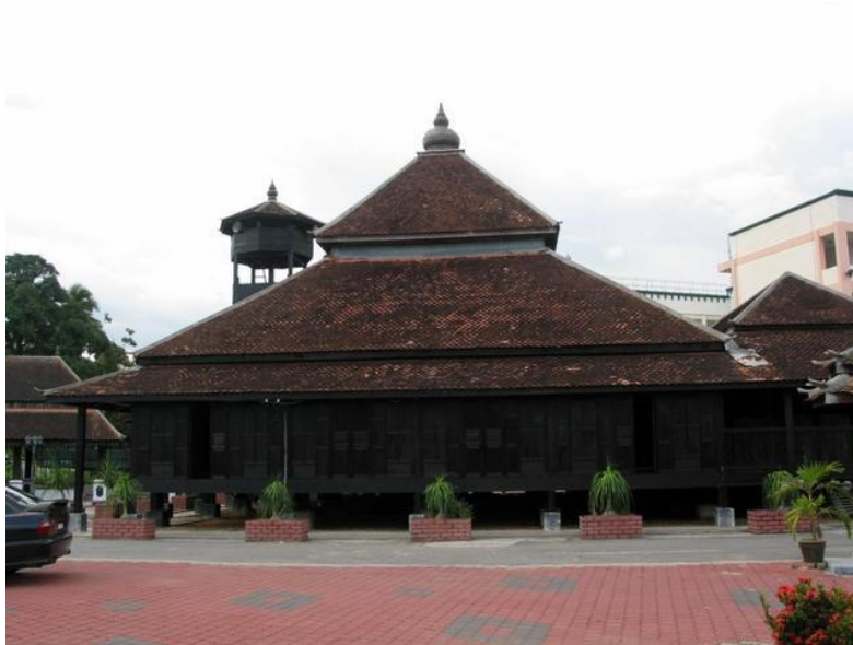
Figure 2. 6 - Picture of Masjid Kampung Laut, Malaysia
