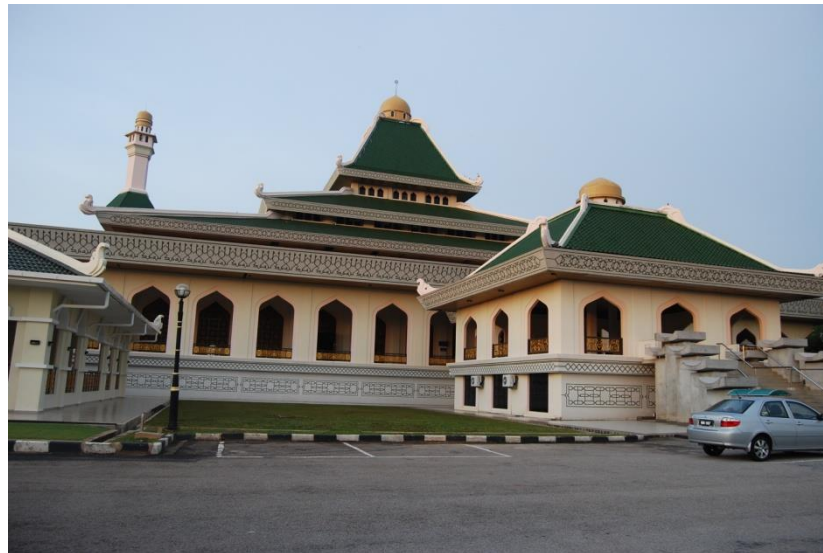
Figure 4. 5 - The side view of Al Azim Mosque, Melaka
