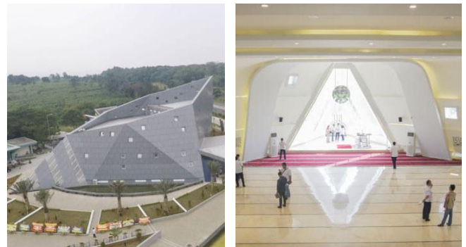
Figure 3: Exterior and interior of Al Safar mosque. Wall composed by triangle composition using ACP. The mihrab area with day light comes from left and right side window
