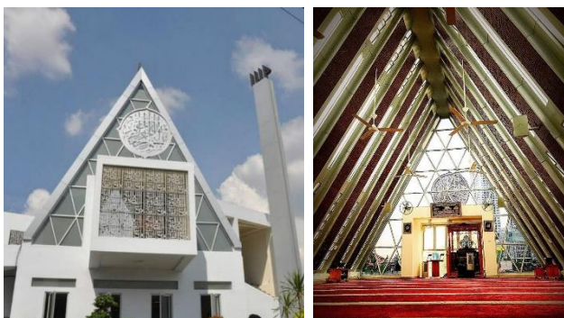
Figure 2: Exterior and interior of Darussalam mosque with A-frame construction that is triangle shape. A-frame construction created isosceles triangular prism interior. The cantilever box is mihrab area.
