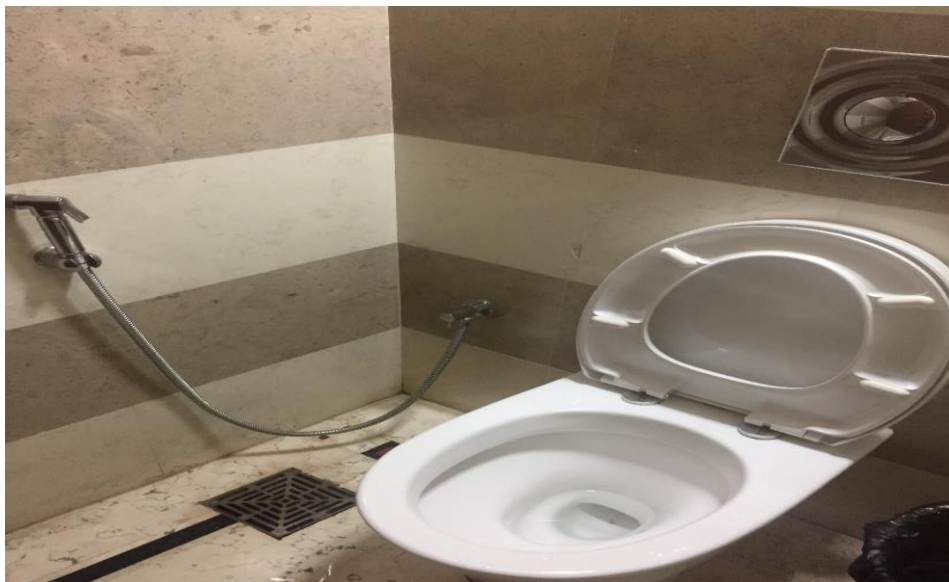
Figure 4.2: Appliances inside the toilet: W/C flush toilet and water tap in the first mosque (Jame)
