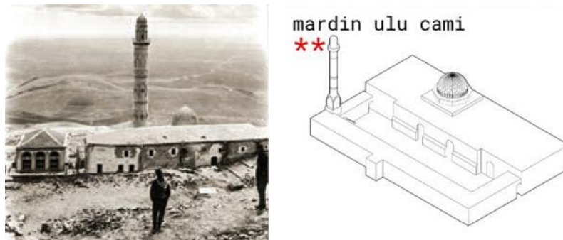
Image 13. The hipped roof of the Mardin Great Mosque in 1911 (Gertrude Bell Archive) (left) Figure 7. Today's flat roof (URL 4) (right)
