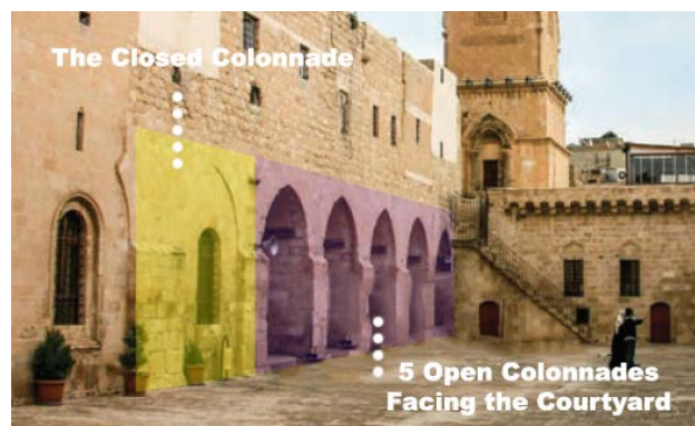
Image 2. Open cloisters and closed cloisters facing the courtyard
