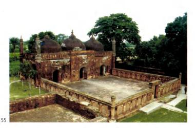
niche from outside, the *kibla* wall is projected in the centre towards the west. The four corners are buttressed by four corner turrets. The turrets are octagonal shaped up to the top of the parapets and then are circular in shape. They are extended high above the roof level and ended in small ribbed cupola having a finial.
