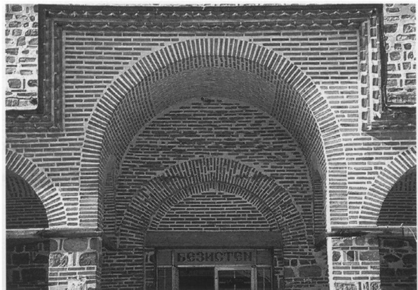
Principal iwan, detail of stone and brick re-pointing
