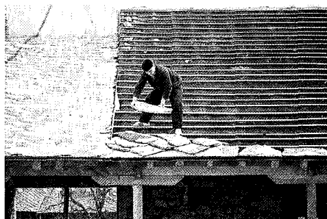
Mostar Old Town: re-roofing a building with the traditional stone
