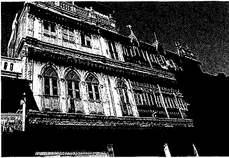
A nineteenth century house with elaborately carved woodwork on the façade in the walled city of Ahmedabad in India. The two top storeys were added later and they should be accepted as part of the history of the building in any restoration programme.
