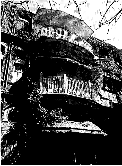
This house in Colaba, Bombay, has characteristic balconies with sun canopies which need protection and control
