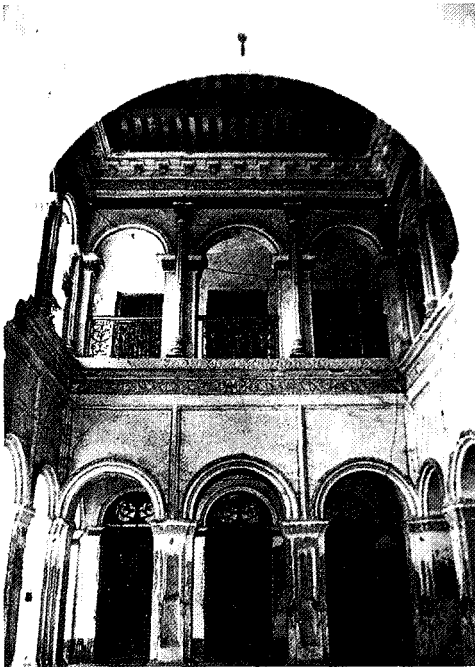
Building #38 exhibits a beautifully-proportioned interior ball with mezzanine.
