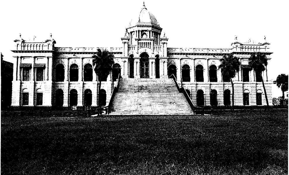
Absan Manzil in 1989, renovated to the 1904 plan Elevation from the river front
