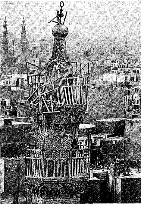
Cairo – Rapid deterioration of the woodwork of a minaret due to neglect
