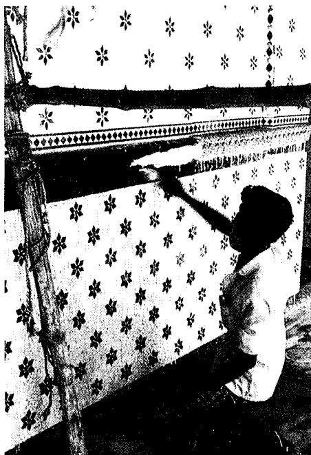
Star Mosque, showing restorer at work and close-up of stars made with broken china pieces
