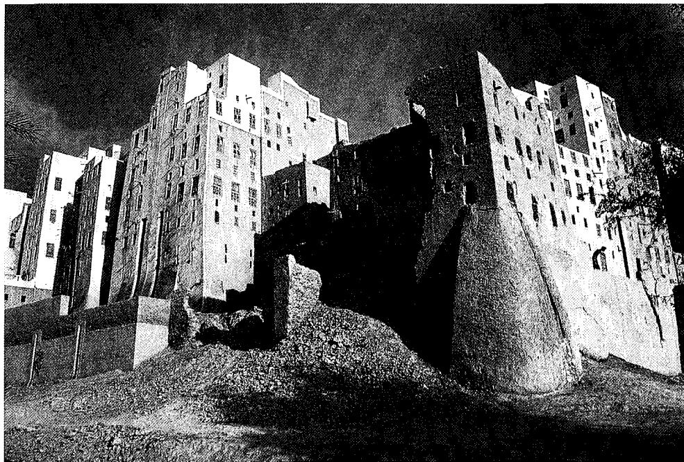
Shibam, Hadramaut – The collapse of the city wall, due to neglect, brought down with it the corner barracks.
