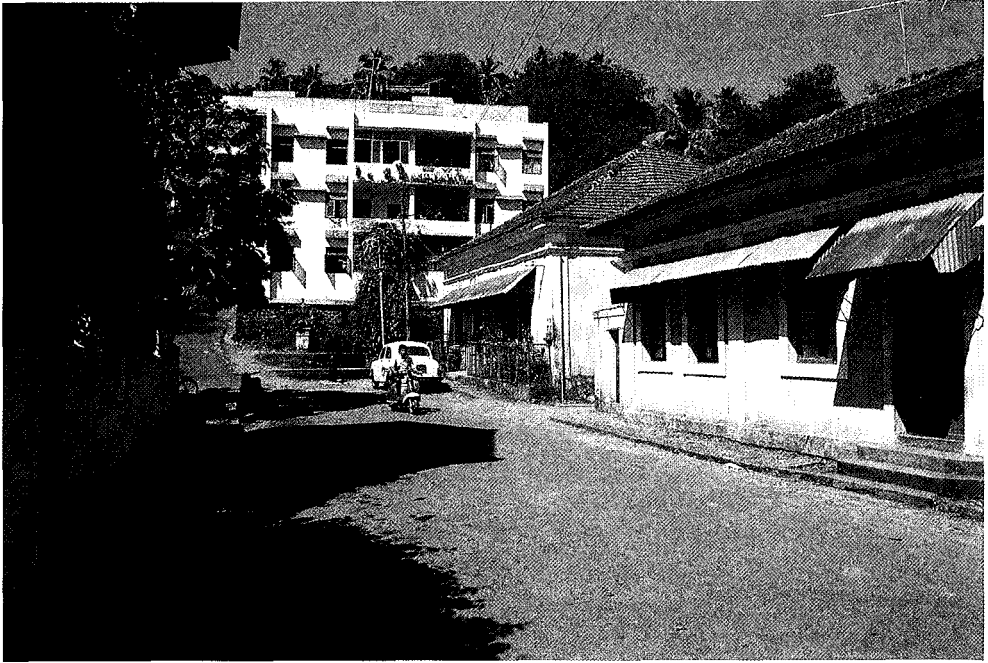
Despite the near conservation area status that Fountain has in Panjim, Goa, this block of flats was allowed in an area which is mainly one- and two-storeys high
