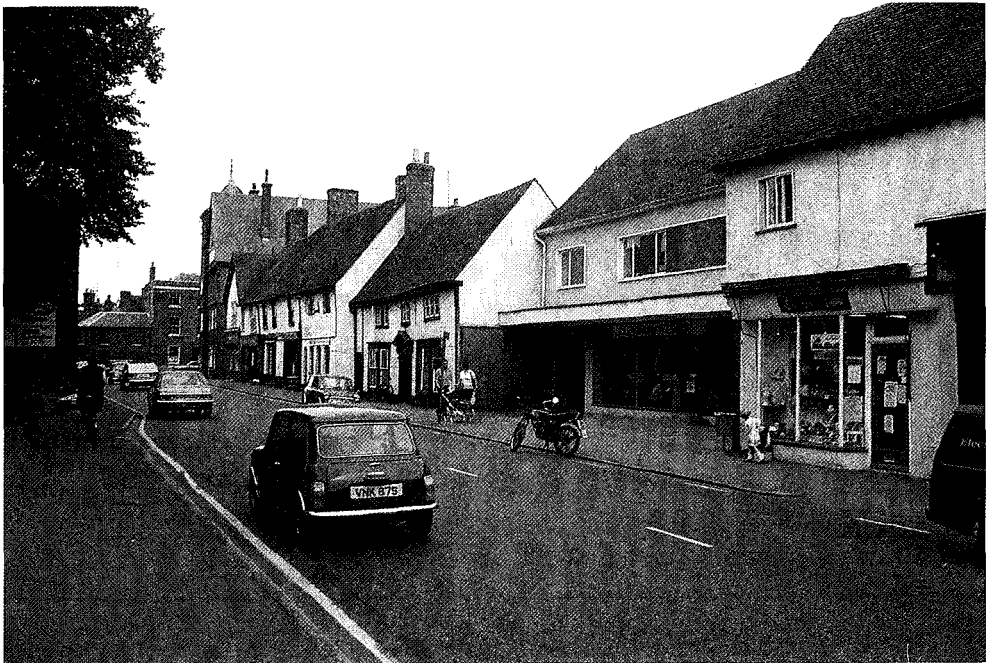
Baldock, Hertfordshire, England: an example of the old and largely discredited practice of setting a new building back from the traditional street frontage in anticipation of overall road widening as the other properties are demolished and rebuilt
