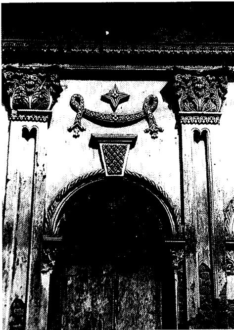
Façade detail showing the elegance of the surface decoration as well as the damage caused by rising damp
