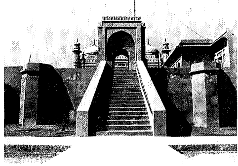
The flight of steps leading up to the gateway entrance of the Mosque
