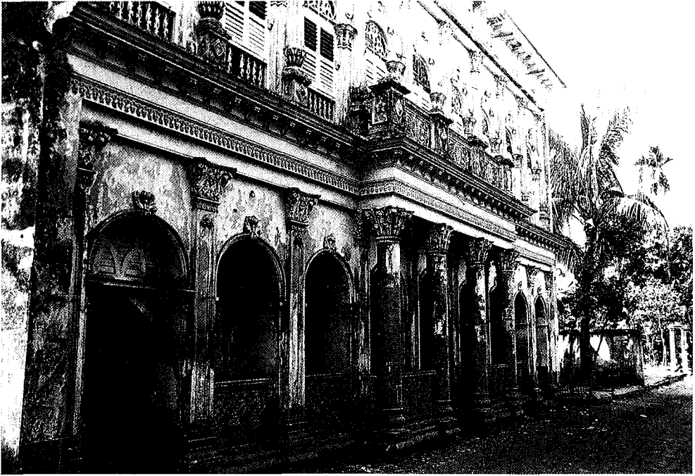
Building #2, proposed for renovation into a hotel, will not need extensive work
