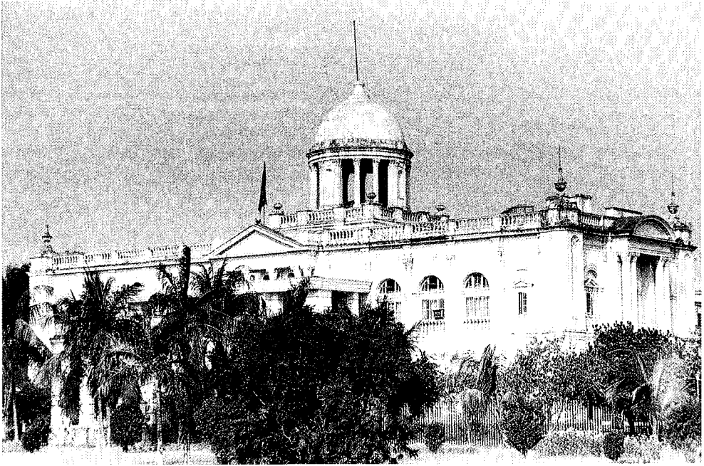
Old High Court Building, view after restoration. Built in 1905 as a governor's residence
