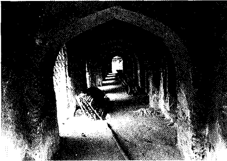
The corridor connecting the cell-like chambers beneath the Mosque's podium
