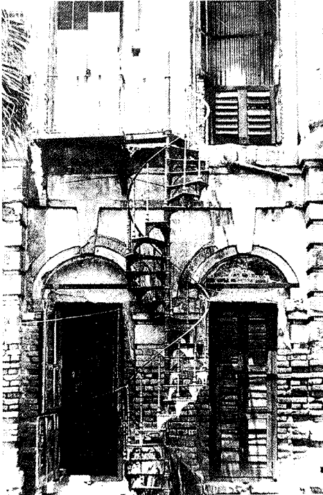
Pre-renovation view of Ahsan Manzil from the east showing the cast-iron spiral staircase used for service access to toilets.
