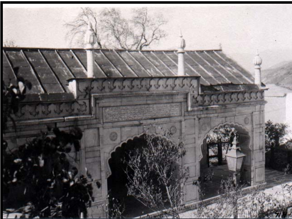
The first documented roof addition, possibly to prevent water seepage, 19 th century.
