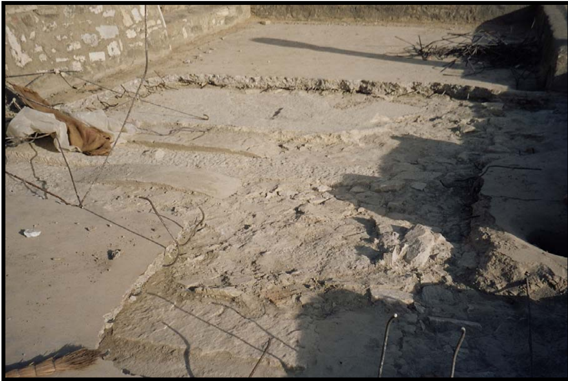
Concrete removal in progress, using hand tools and after the erection of shuttering to provide additional support to the roof.
