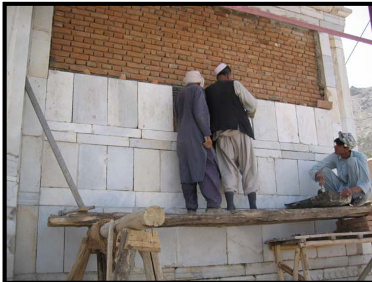
Marble facing being built into the new brick wall.
