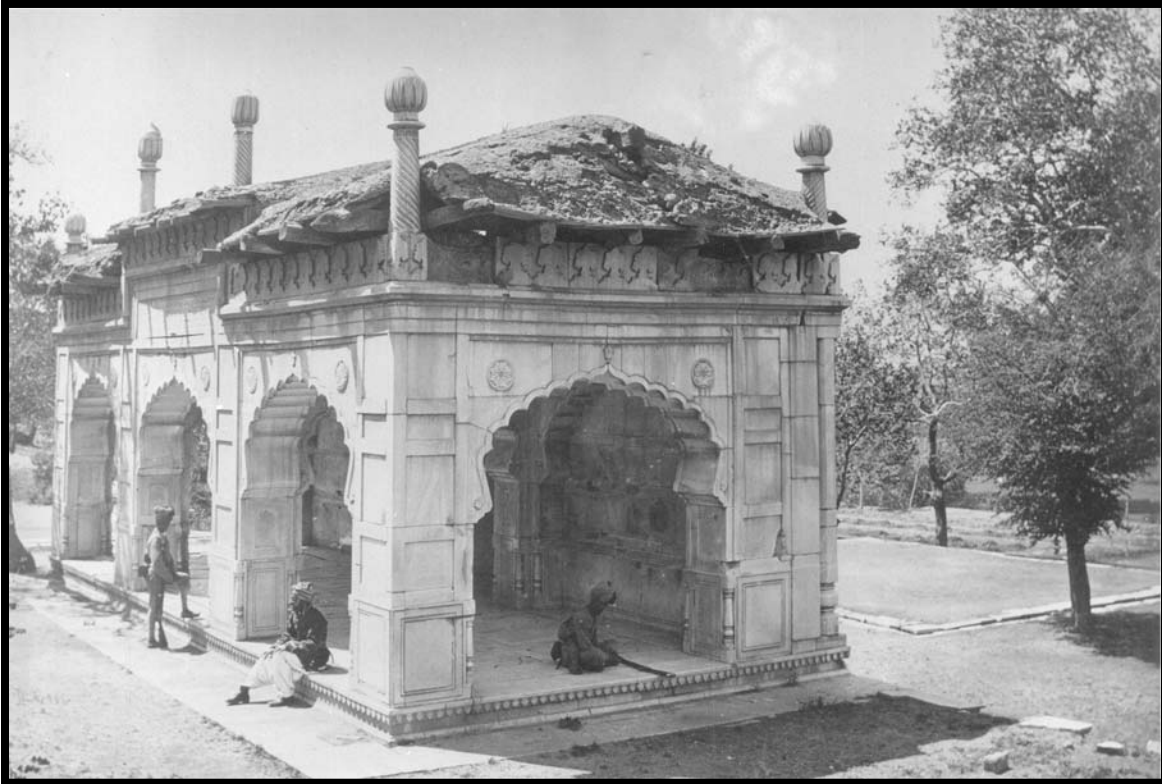
The first documented roof addition, possibly to prevent water seepage, 19 th century.
