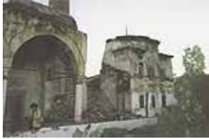
The Hadum Mosque complex: the madrasa (right) has already been demolished, and the mosque (left) is still under threat
