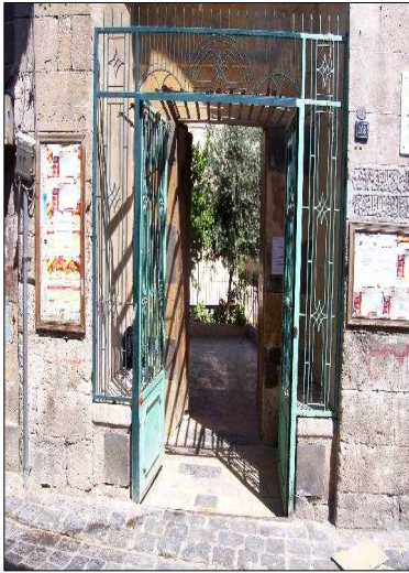
Plate (2) Lower part of the main entrance
