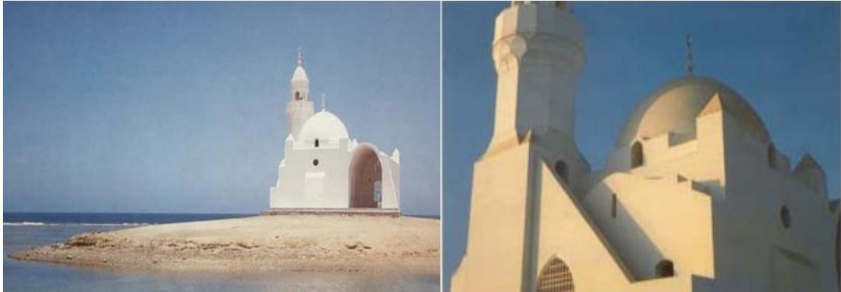
Figure 6.8: The Corniche mosque overview and a close up to its geometric architectural forms.
