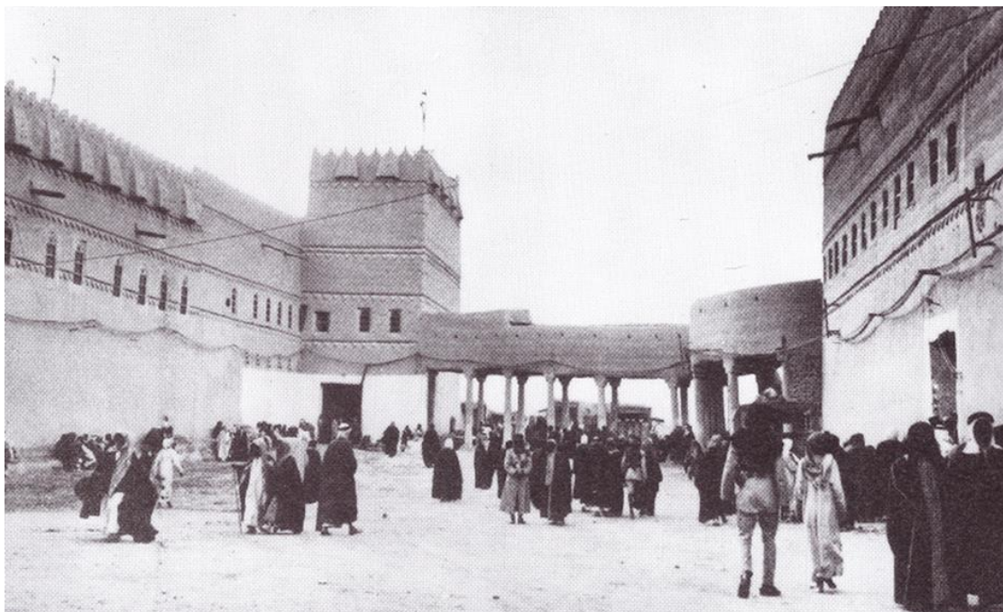
Figure 7.26: The front of the palace from the palace square in 1935. Source: (Facey, 1992, p.282).
