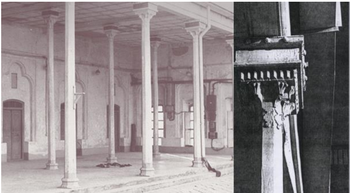
Figure 8.14: The columned porch and the arches. Source: (Lewcock and Freeth ,1978, p.72), and a close look at the column capital details. Source: (Kuwait municipality publications, 1986).
