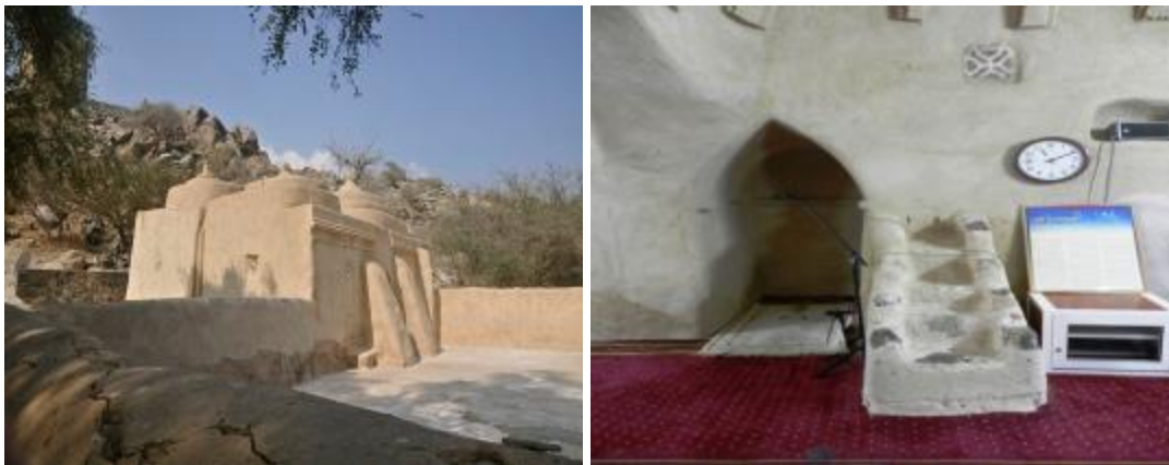
Figure 4.7: Al Badiyah Mosque in Fujairah city. To the right are the mihrab and the minbar.
