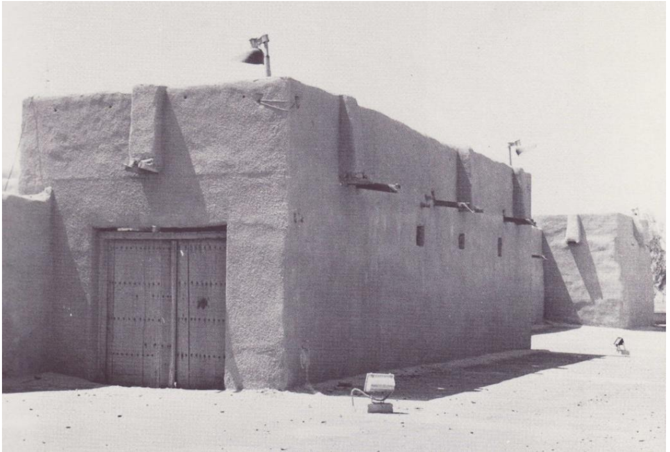
Figure 8.21: Entrance gate to the red fort. Source: (Lewcock and Freeth, 1978, p. 81).
