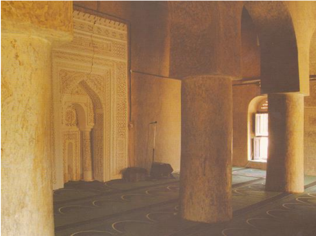
Figure 8.53: View of the mihrab of the Musimat mosque, showing the decorative gypsum work and the central column in the prayer hall. Source: (Al-Salimi et al., 2008, p. 65).
