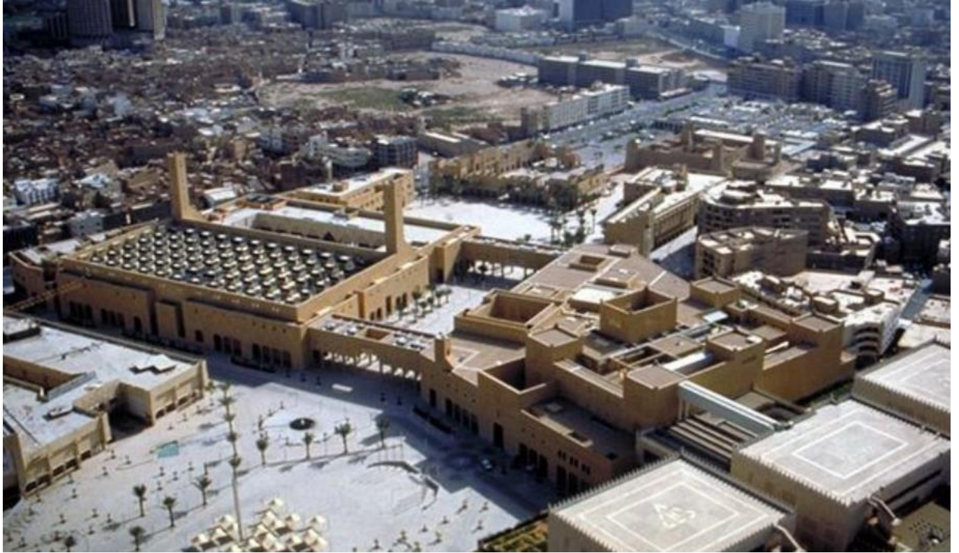
Figure 7.30: Aerial view of the Qasr Al-Hkoum mosque at the left, with the palace at the right.
