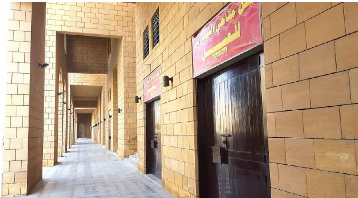
Figure 7.34a: wall-arcades with shop units opening to the north road. Source: (Photos commissioned by the author).
