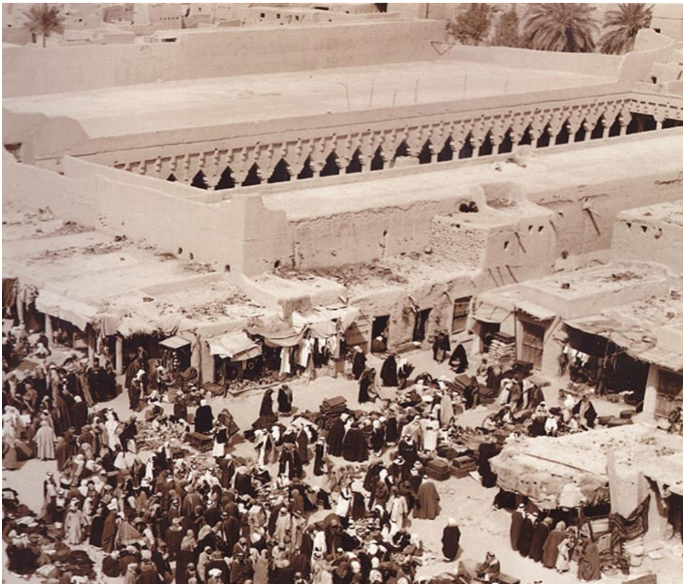
Figure 7. 24: A photograph of the marketplaces/shops attached to the mosque and the main square, in 1949. Source: (The High Commission For the Development of Ar-Riyadh publications, 2006, p. 16).
