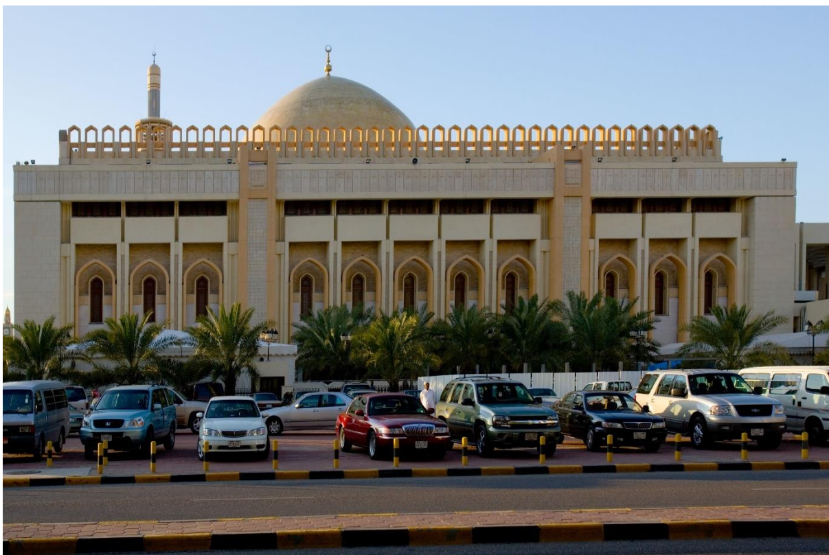
Figure 8.31: South view of the mosque, showing the additional car park space and tents at the back. Source: (ibid).
