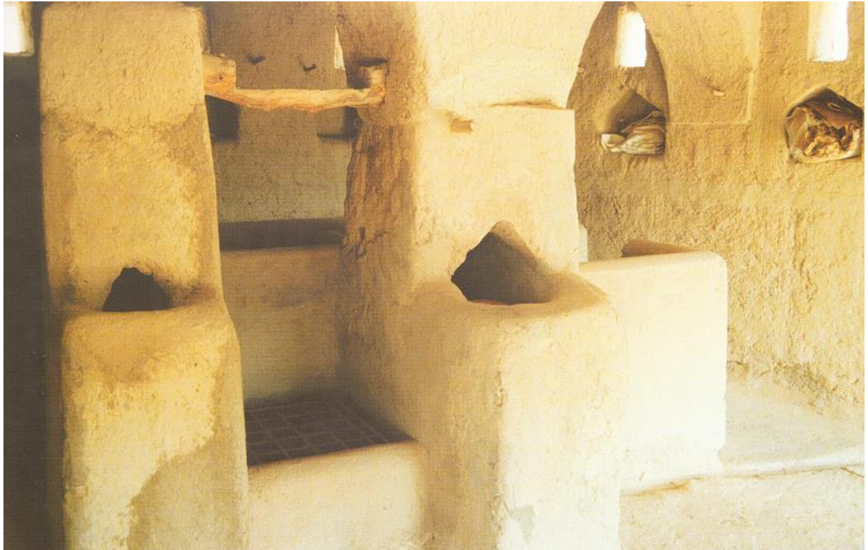
Figure 8.48: Ablution area at Bahla mosque, with falaj running underground. Source: (Al-Salimi et al., 2008, p. 81).
