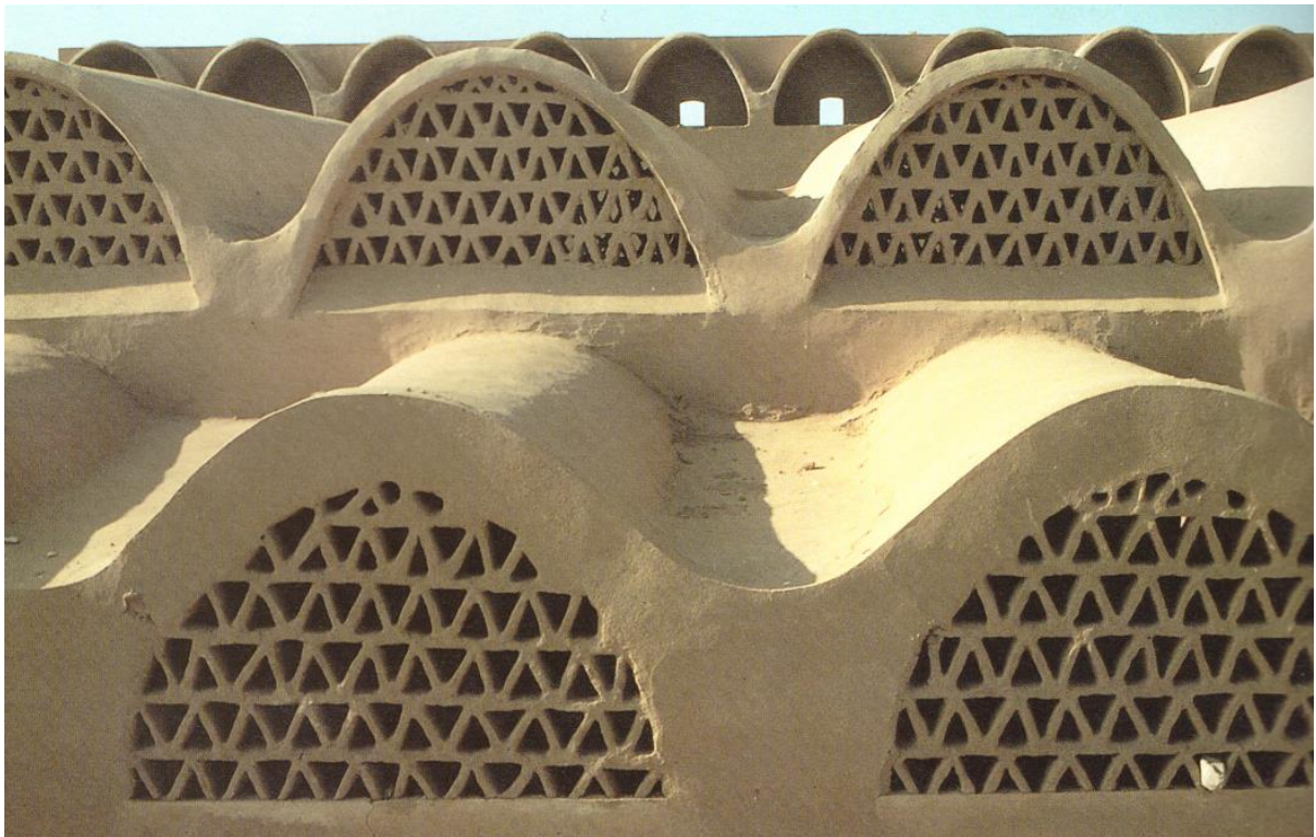
Figure 6. 18: Souk, New Bariz, Egypt, 1967, air inlets. Source: (Steel, J, 1988, p. 16).
