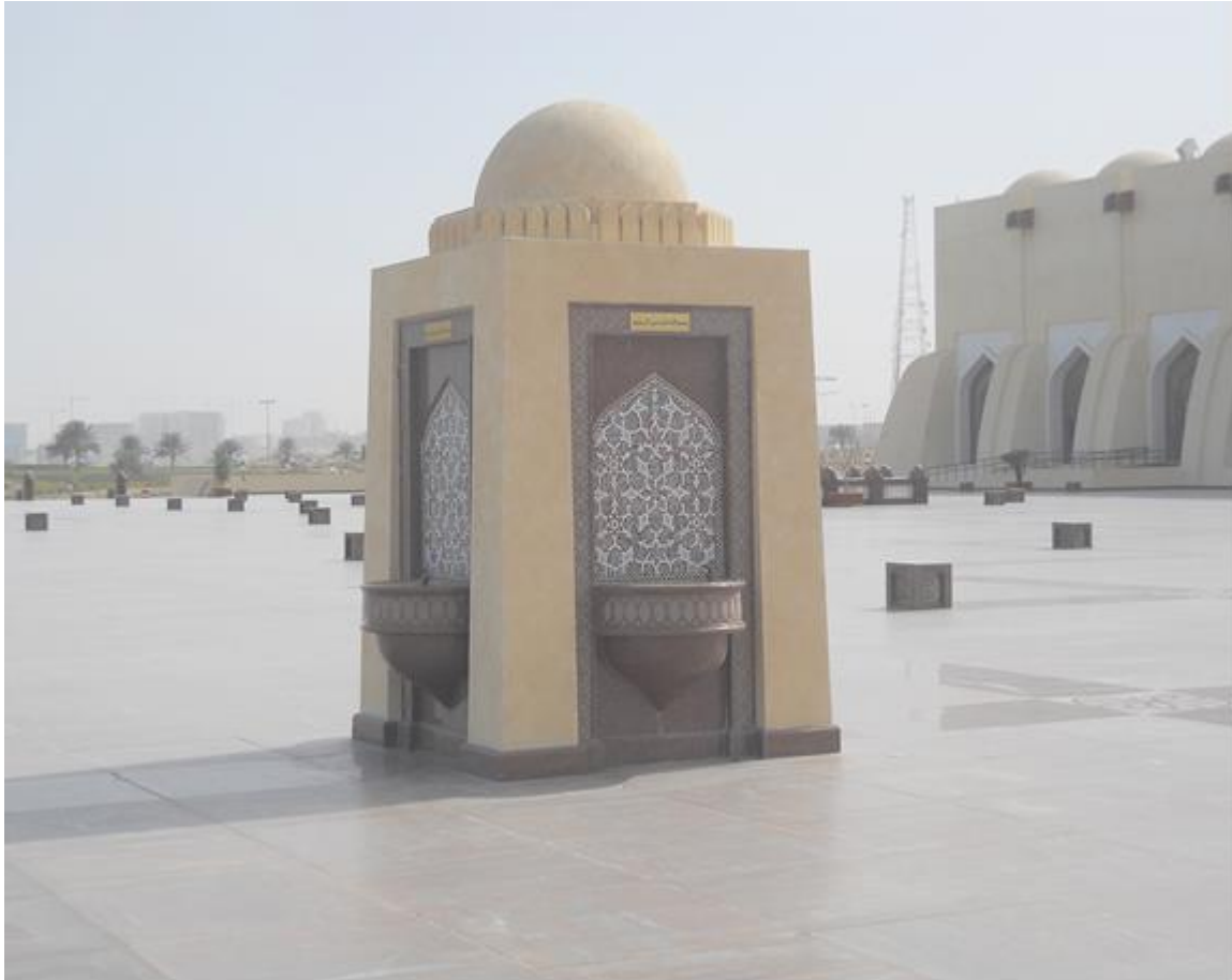
Figure 5.12: The drinking water fountain unit positioned at the front courtyard. Source: (ibid).
