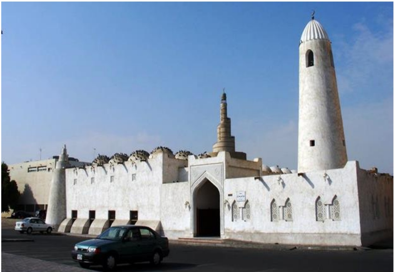
Figure 5.6: Al Qubib Mosque in Doha restored in 2012. Source: (publications ministry of Islamic affairs of Qatar).
