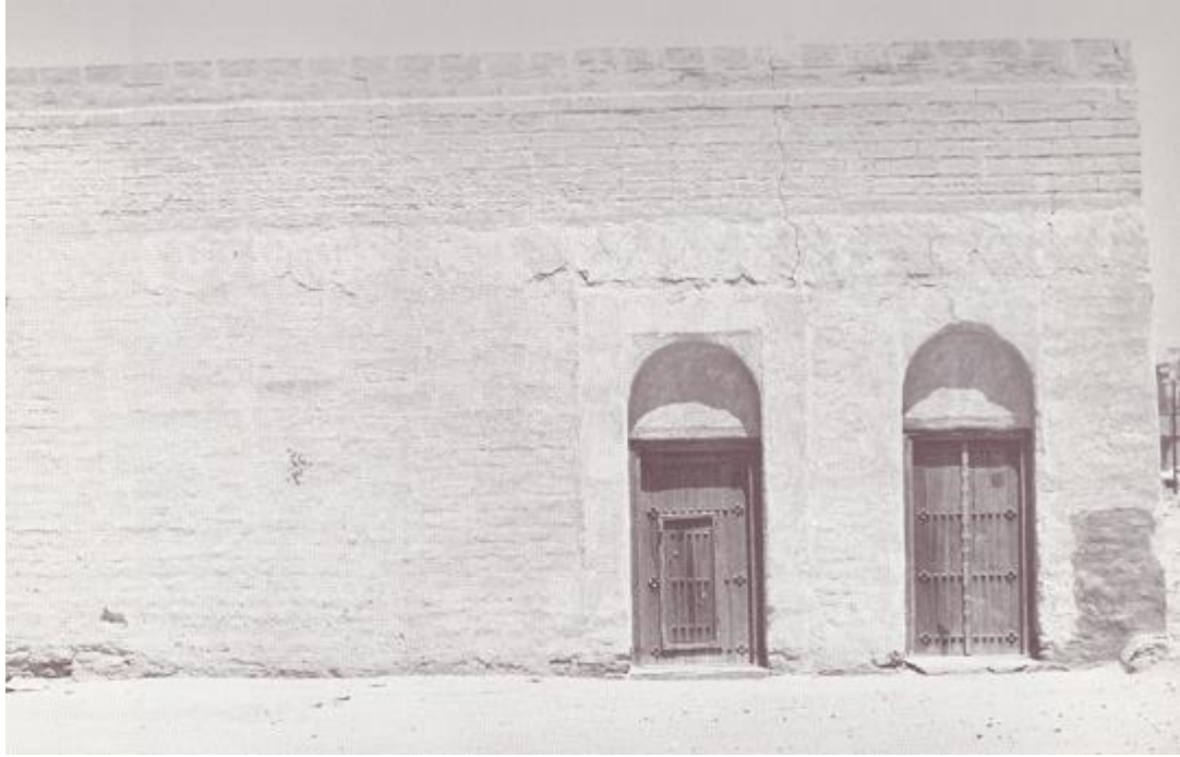
Figure 8.15: Typical façade of an old house in Kuwait; rounded niched arches framing doors.
