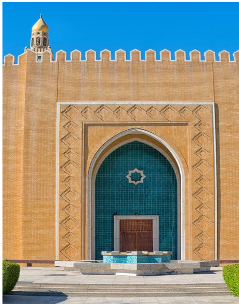
Figure 8.18: View of the portal arch from inside the palace. Source: (commissioned by the author).
