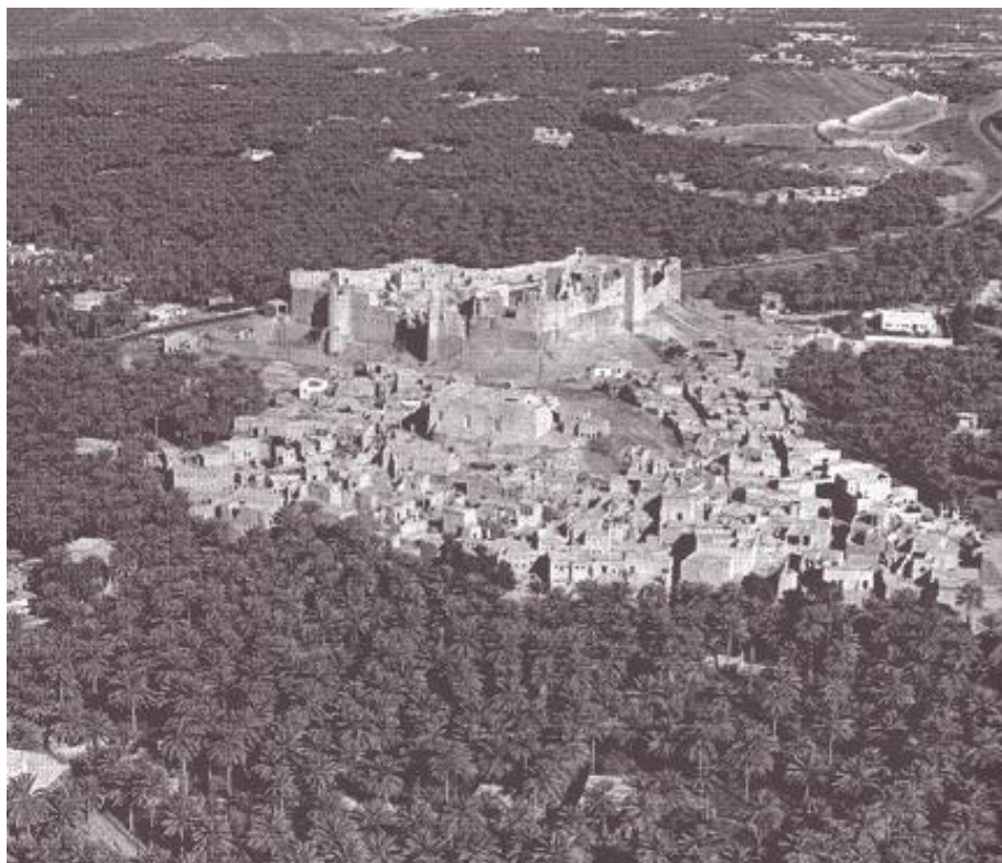
Figure 8.63: View of Bahla with the citadel in the centre with residential quarter and the mosque in the foreground. Source: (Costa, 2001, p. 74).
