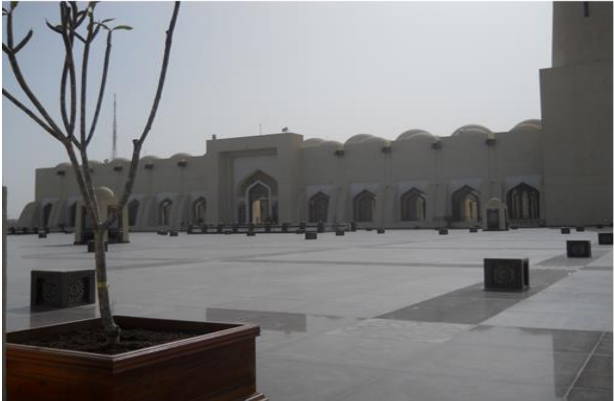
Figure 5.10: The main gate and the front courtyard. Source: (ibid).
