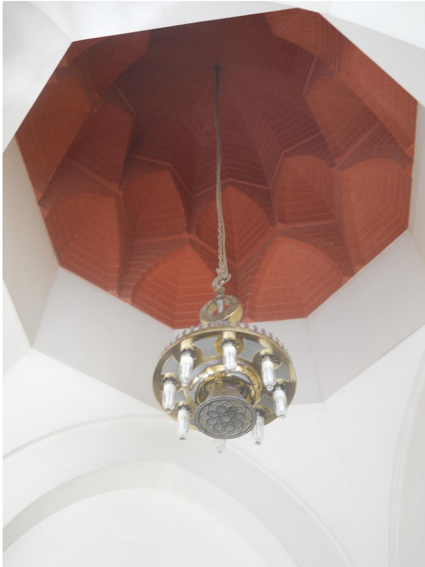
Figure 6.25: the interior of the dome showing the red bricks and the chandelier. Source: (ibid).
