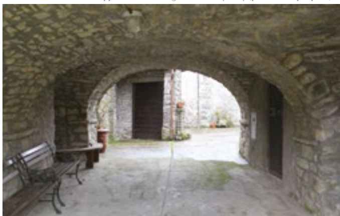
Fig. 9 Stone masonry vaults increase the mass of the building at the ground floor and create a solid connection between opposed walls. Lunigiana, Tuscany, Italy (photo: L. Dipasquale).
