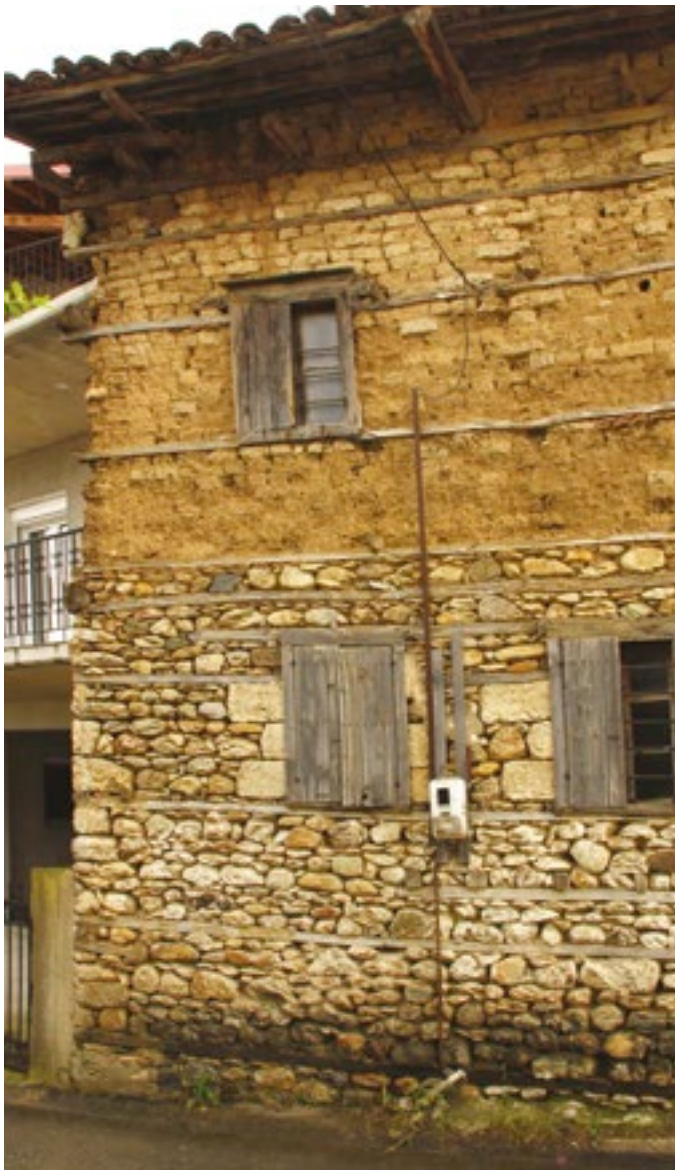
Fig. 13 Stone and adobe building with hooping reinforcement in Kastaneri, Greece (photo: S. Mecca).
