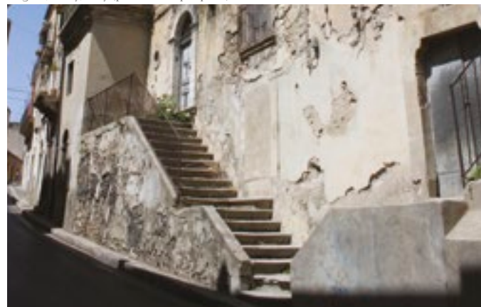
Fig. 10 External staircases lower the centre of gravity of the building and reinforce its base Ragusa, Sicily, Italy (photo: L. Dipasquale).
