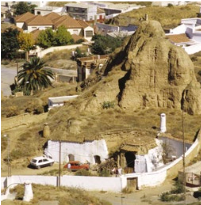
Fig. 1 Cave dwelling excavated on the slope of a promontory in Guadix, Spain (photo: F. Vegas and C. Mileto).
