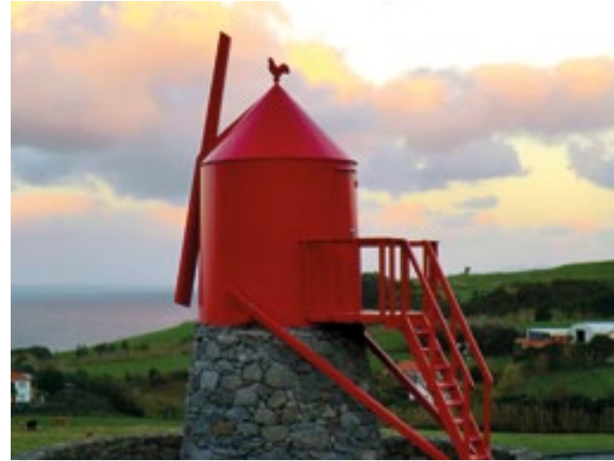
Fig. 8 Energy management: a windmill in the island of Faial, Azores, Portugal (photo: M. Correia).
