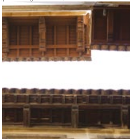
Fig. 1 Eaves in a street of Palma de Mallorca preventing the sun from impacting on façades and streets. Spain (photo: F. Vegas, C. Mileto).
