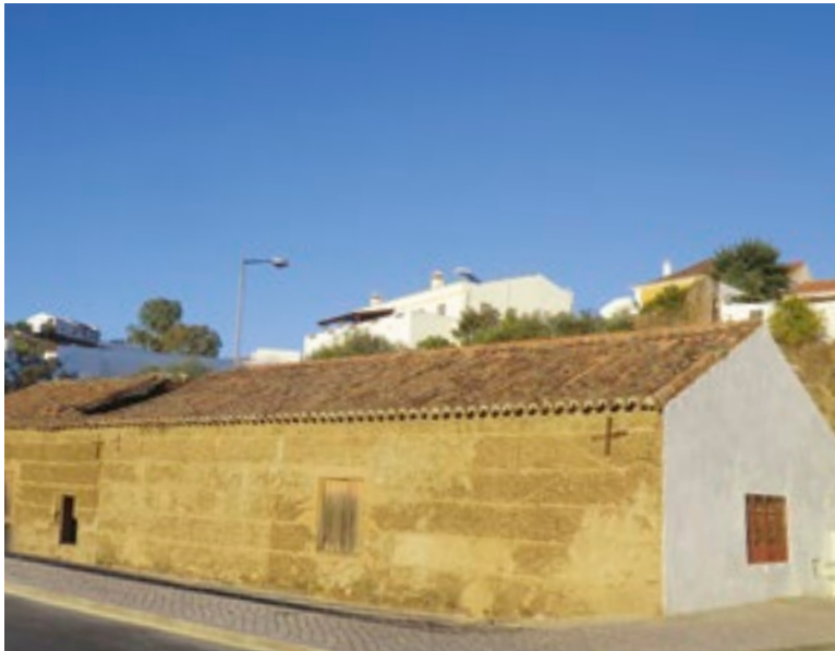
Fig. 5 Rammed earth building in Mértola, Alentejo, Portugal (photo: M. Correia).
