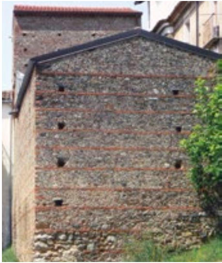
Fig. 1 Rows of bricks used for wall reinforcement, Lamezia, Calabria, Italy (photo: L. Dipasquale).
