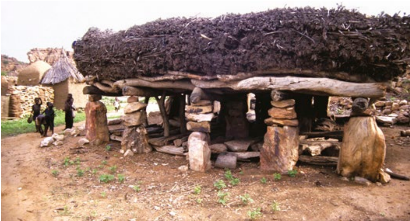
Fig. 9 The toguna of the Dogon people are public buildings built on pillars. Mali (photo: F. Vegas, C. Mileto).
