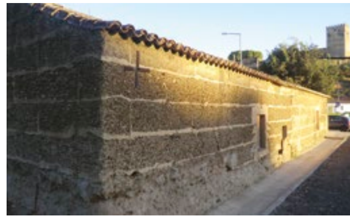
Fig. 5 Anchor plates in a rammed earth building, Mertola, Portugal (photo: M. Correia).
