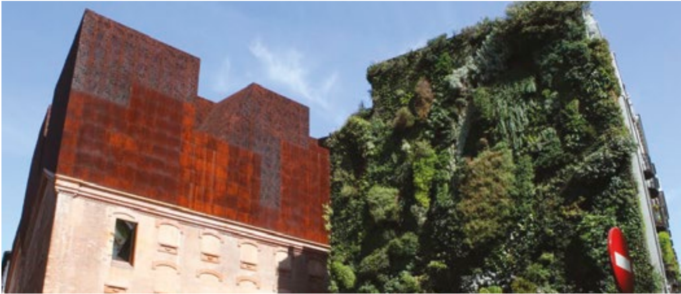
Fig. 3 Caixa Forum building in Madrid by Herzog and de Meuron, with its vertical garden designed by the French botanist Patrick Blanc (2008). Madrid, Spain (photo: L. Dipasquale).
