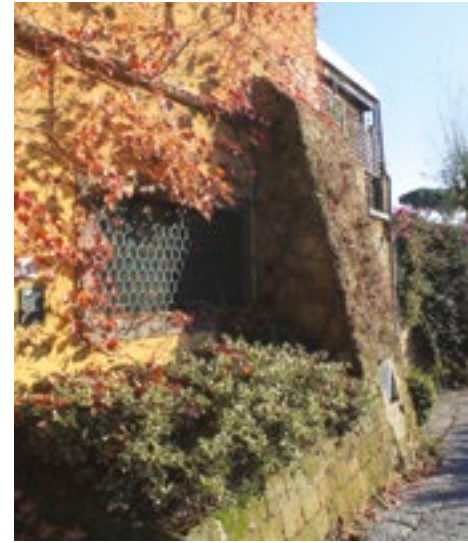
Fig. 3 Butress in a masonry building, Naples, Italy (photo: L. Dipasquale).
