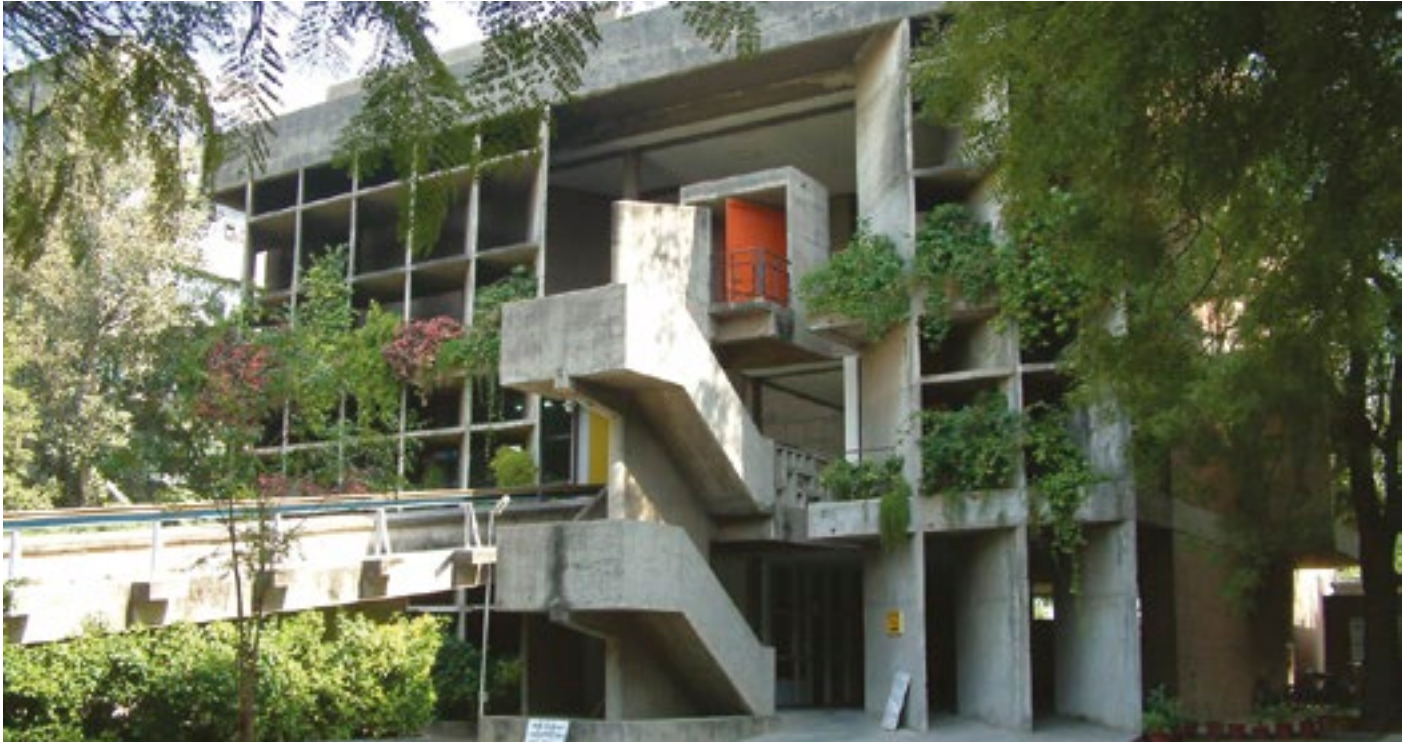
Fig. 23 Millowner's Association building by Le Corbusier, with its characteristics brise-soleils to prevent the hard sun from entering inside. Ahmedabad, India (photo: F. Vegas, C. Mileto).
