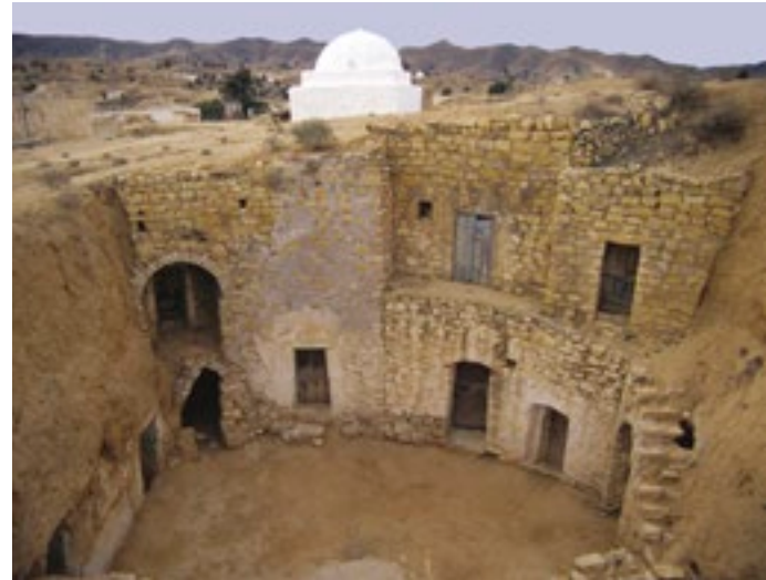
Fig. 10 A cave dwelling with its characteristic patio for an extended family. Matmata, Tunisia (photo: F. Vegas, C. Mileto).
