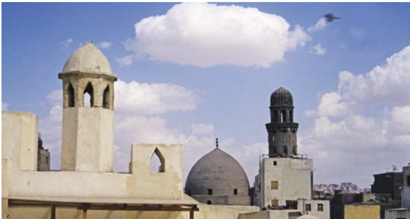
Fig. 22 Vents on top of stairways and domes that generate the circulation and renewal of fresh air in the dwellings. Cairo, Egypt (photo: F. Vegas, C. Mileto).
