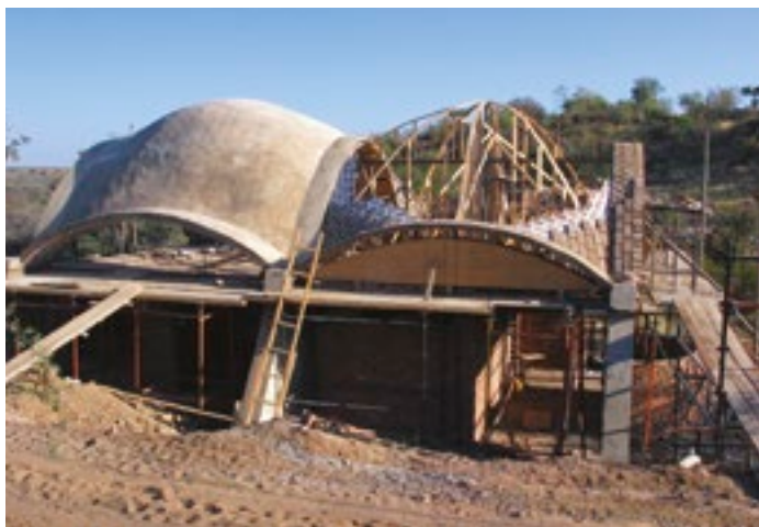
Fig. 11 Mapungubwe Interpretation Centre while being erected with local craft and materials. Limpopo, South Africa. (photo: J. Bellamy)
