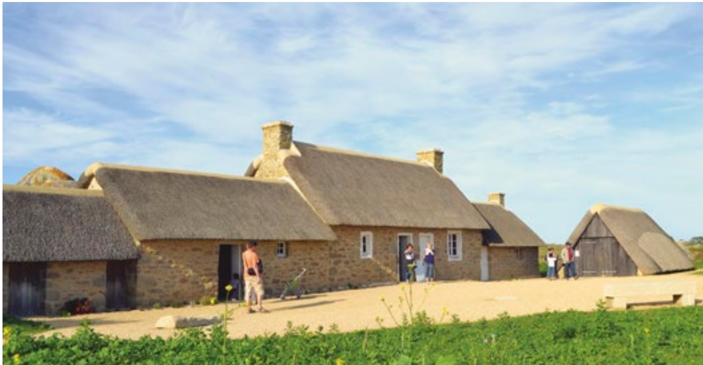
Fig.8 Thatched roofs in the fishermen's village of Meneham, Bretagne, France (photo: H. Guillaud).
