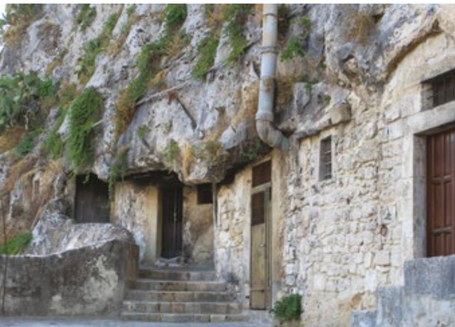
Fig.2 Underground dwellings in Scicli, Sicily, Italy.
