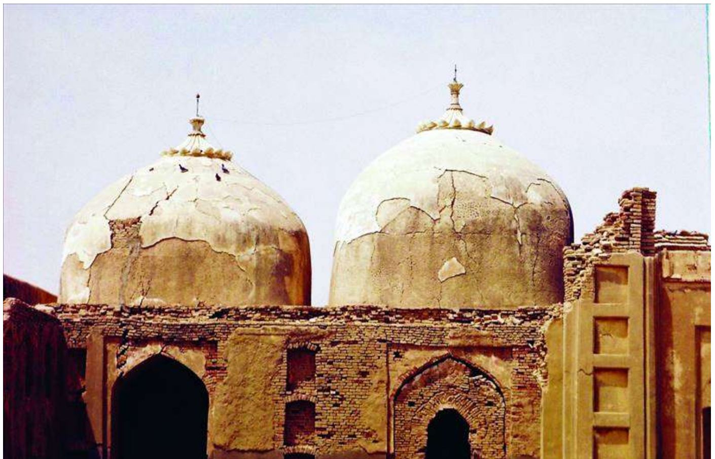
Closer view of mosque domes
