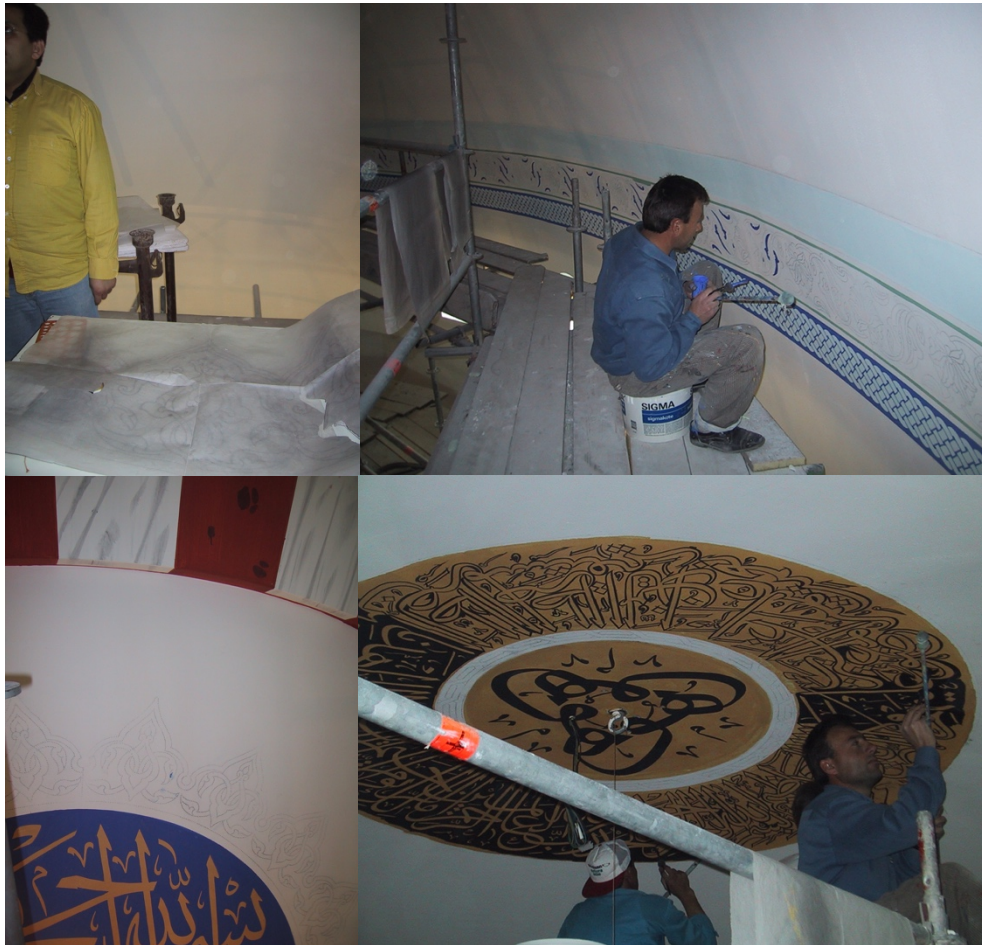
Fig. 19. Process of how the decorations are made on the dome, walls and columns (Toorman Architecture Archive, 2021)
