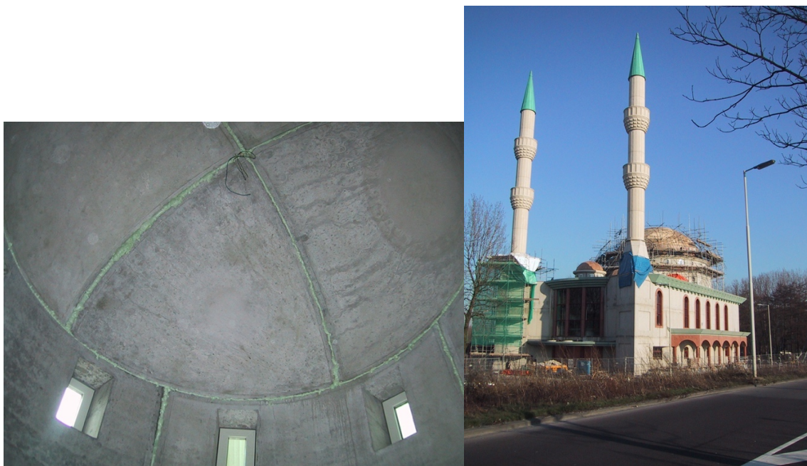
Fig. 15 and 16. The construction of the dome consist of prefab concrete. The concrete dome is topped with a wooden structure to connect the patinated copper. Source: (Toorman Architecture Archive, 2021)
