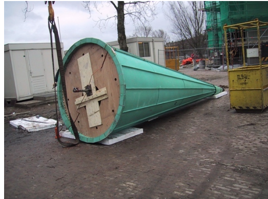
Fig. 23. Wooden structure used for the spire with a patinated copper cladding Source: (Toorman Architecture Archive, 2021)
