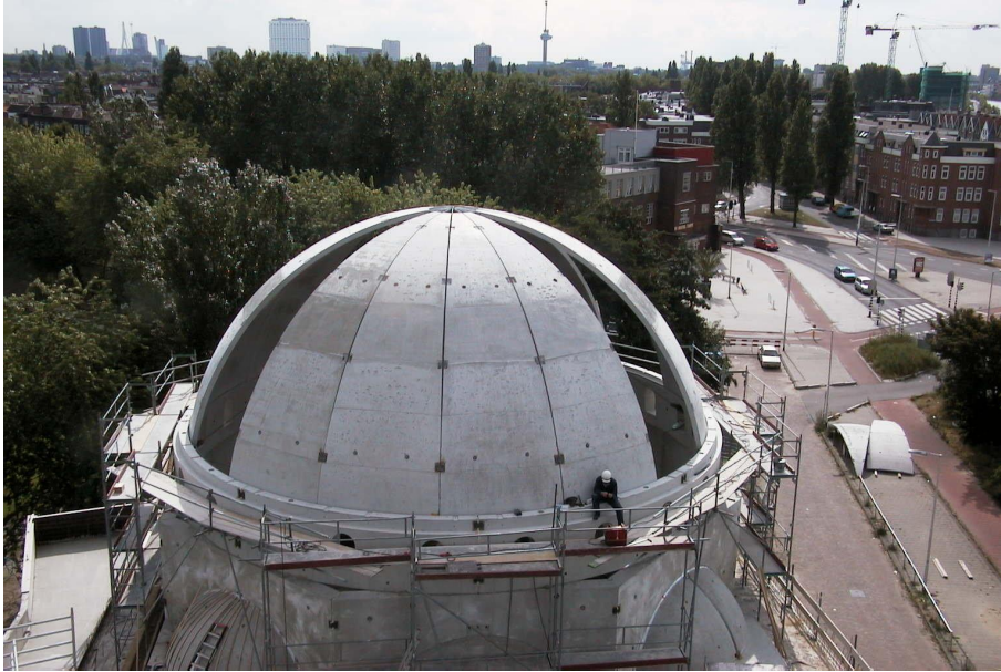
Fig. 14. A birds view of the dome made of several concrete parts. Source: (Toorman Architecture Archive, 2021)
