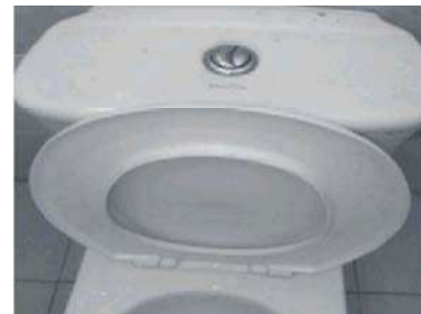
Fig. 3: Application of Double Flushing Cistern for Toilets in Masjid Wakaf Tembesu Kuala Terengganu
