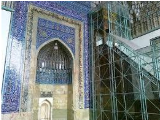
Figure 5. Maqsurah veranda after the reconstruction, Razavi holy, Mashhad, Iran
