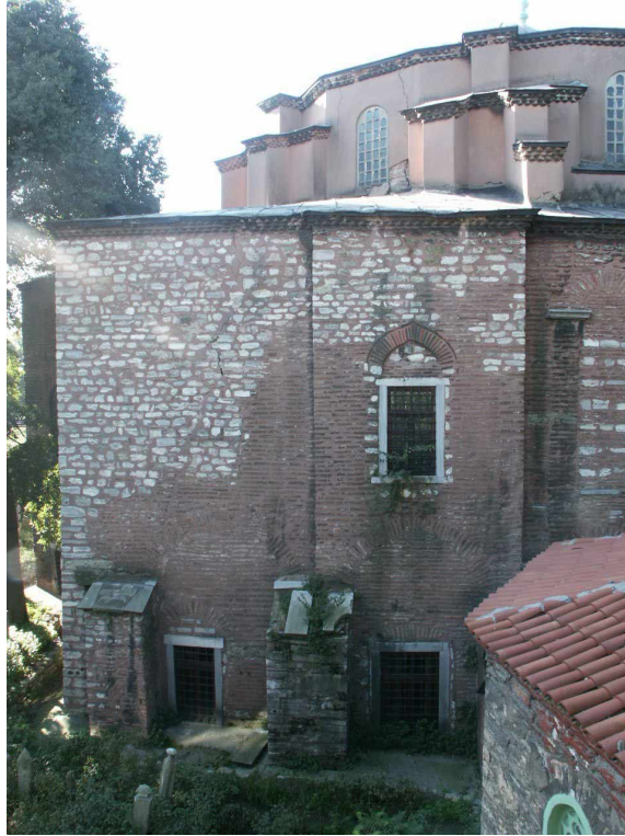
Figure 6 Damaged, rebuilt and strengthened wall parts of the north-east view
