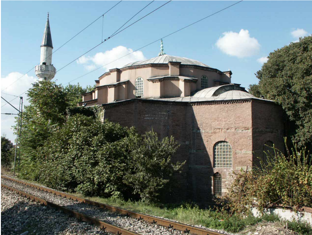
Figure 1 a) General view of the Little Hagia Sophia Mosque and the rail way between the building and the sea.
