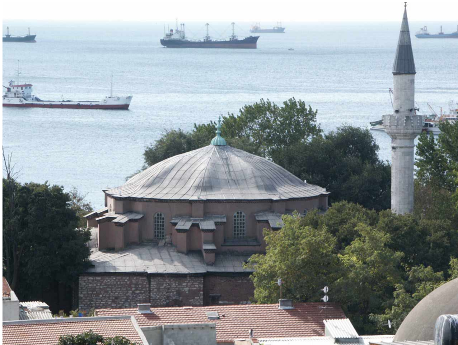
Figure 1 b) General view and the main dome of the Little Hagia Sophia Mosque
