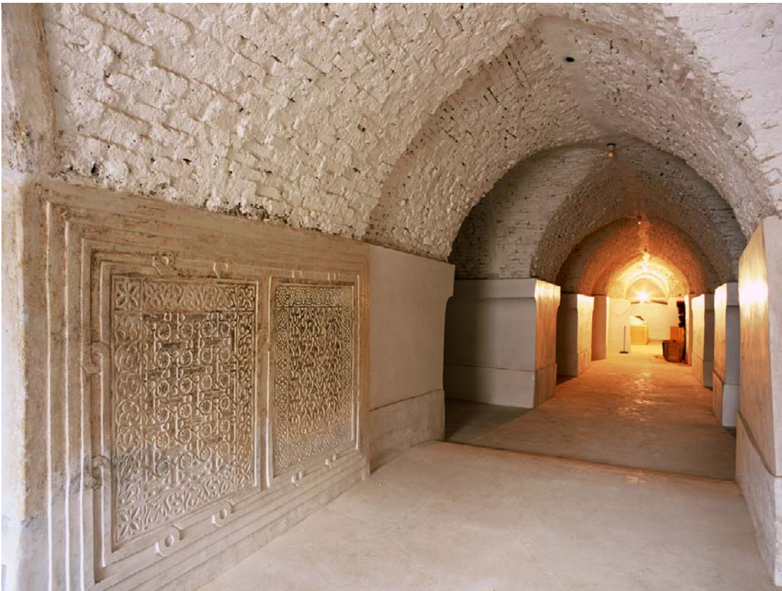
Ground floor corridor after restoration, with carved quadad panels at the lower left.
