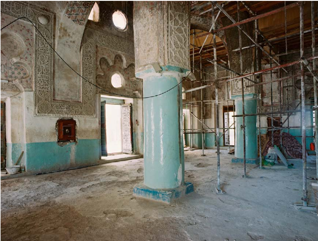
View of the prayer hall during restoration.
