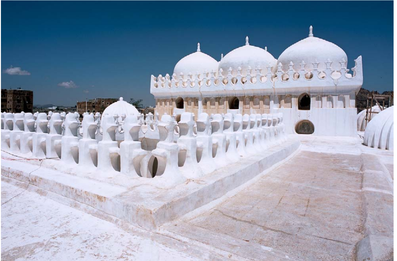
The domes of the masjid are in stone; a double set of clerestory alabaster windows is set in the platform from which the domes rise.
