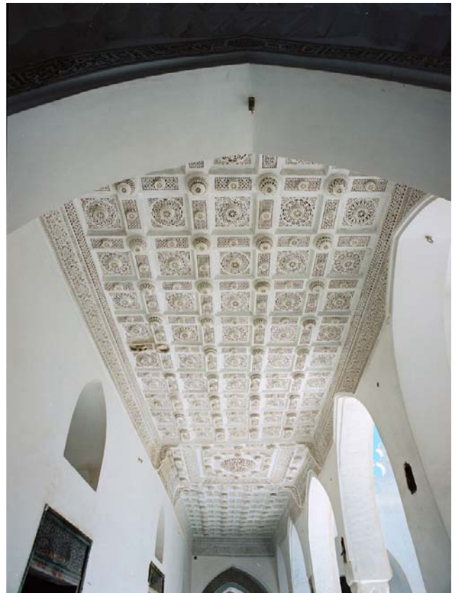
Detail of the stuccowork in the coffered ceiling in the gallery surrounding the courtyard.
