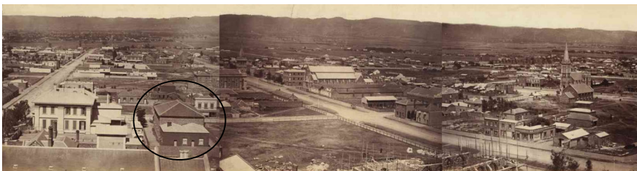
Fig. 2 View of Adelaide from the Town Hall Tower, looking east, identifying the Freeman Street Congregational Chapel ( circle ). Townsend Duryea, 1865. State Library of South Australia B5099/4, B5099/5 and B5099/6 (composite image by author). (No known copyright restrictions)
