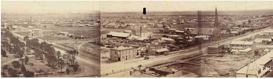
Fig. 3 View of Adelaide from the Town Hall Tower, looking south west, identifying the approximate location of the Adelaide Mosque which was begun in 1889 ( arrow ). Townsend Duryea, 1865. State Library of South Australia B5099/9, B5099/10 and B5099/11 (composite image by author). (No known copyright restrictions)
